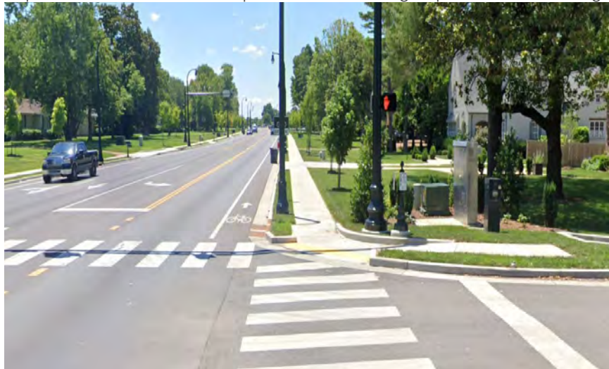
Existing bicycle lane on Hillsboro Road.
