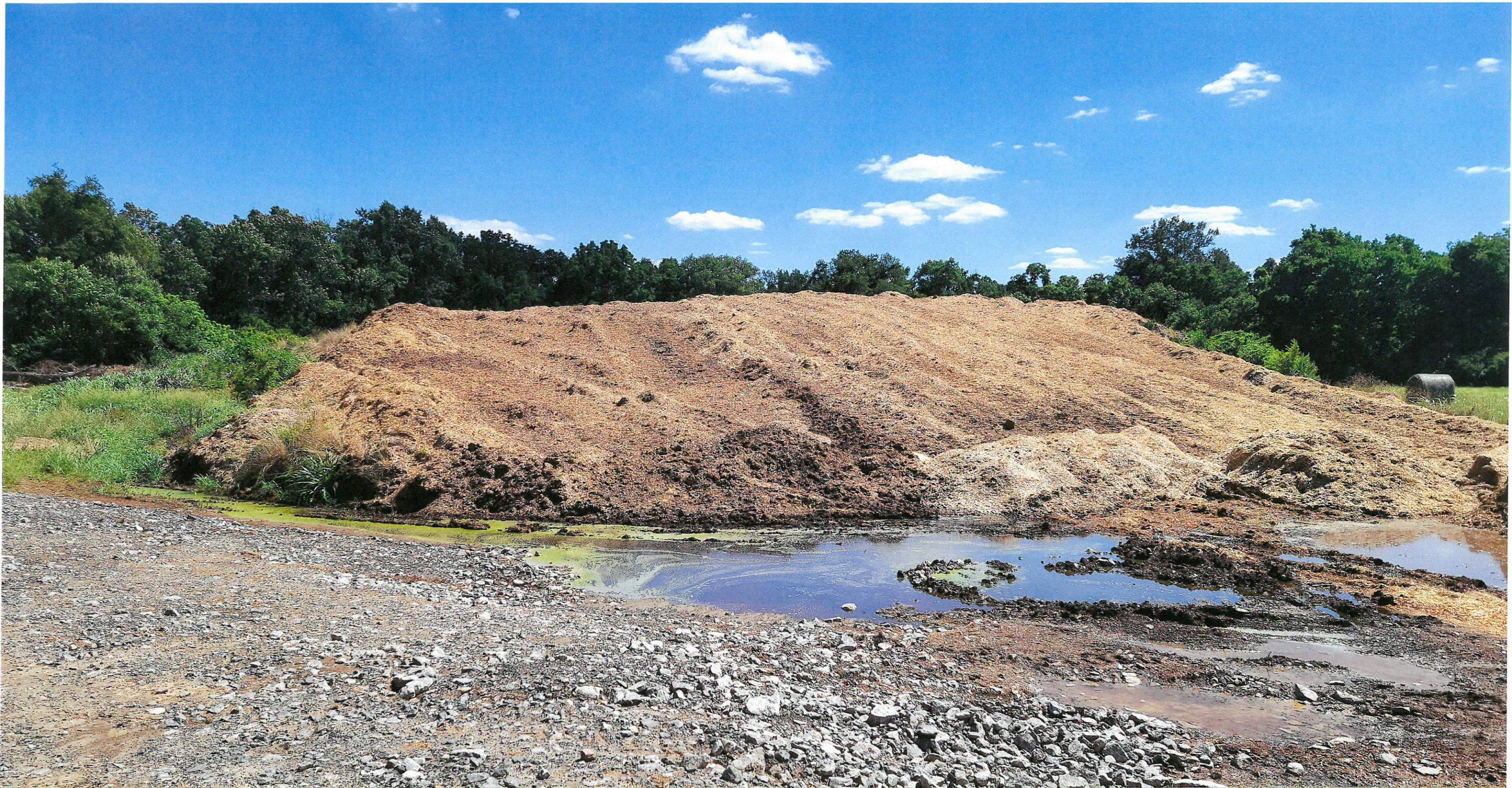
EXISTING MUCKED STALL DISCARD AT SOUTH END OF PROPERTY TO BE REMOVED
