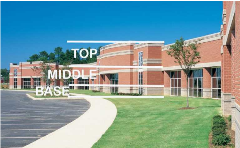
The Schilling Farms Business Center illustrates a clear division of the vertical facade. In the picture, the base is articulated in a differently colored brick, while windows and brick columns characterize the middle, and a band of brick flanked by off white trim separates the top.
