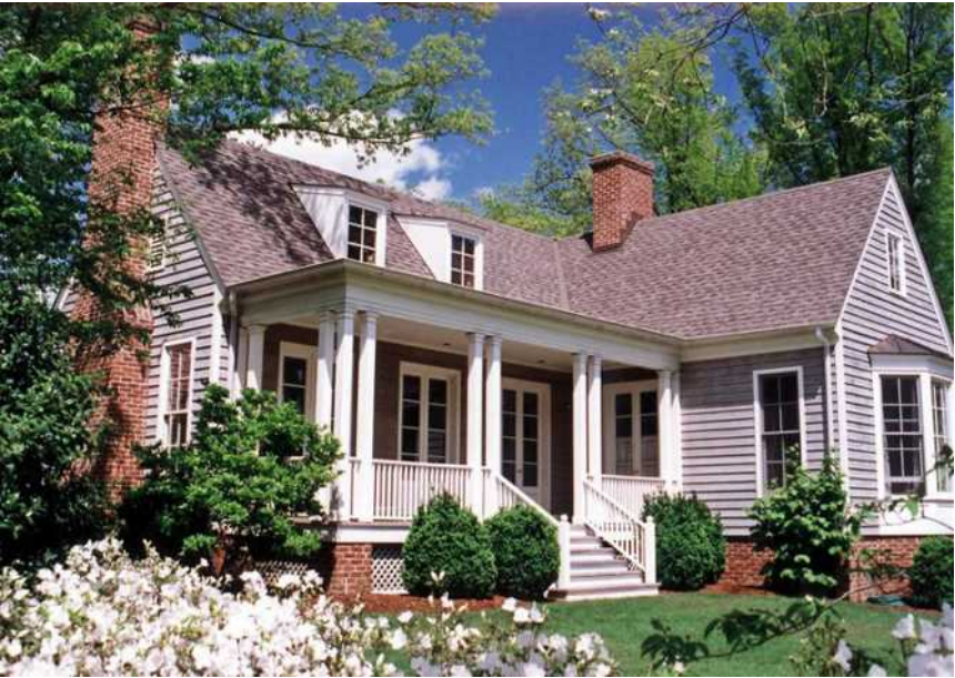
Architect: Oscar Menzer In this example, notice the wood siding, the brick chimneys, and the brick foundation.
