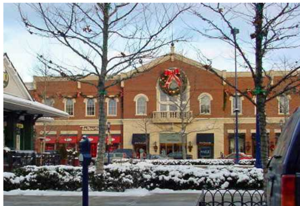
Easton Retail Building, Ohio The Easton retail building (shown left) incorporates a tripartite scheme into its principal facade by emphasizing the central entry. The central section is the most distinctive element on this building because of its dominating size, its protruding nature, and by incorporating a federal-style pediment.
