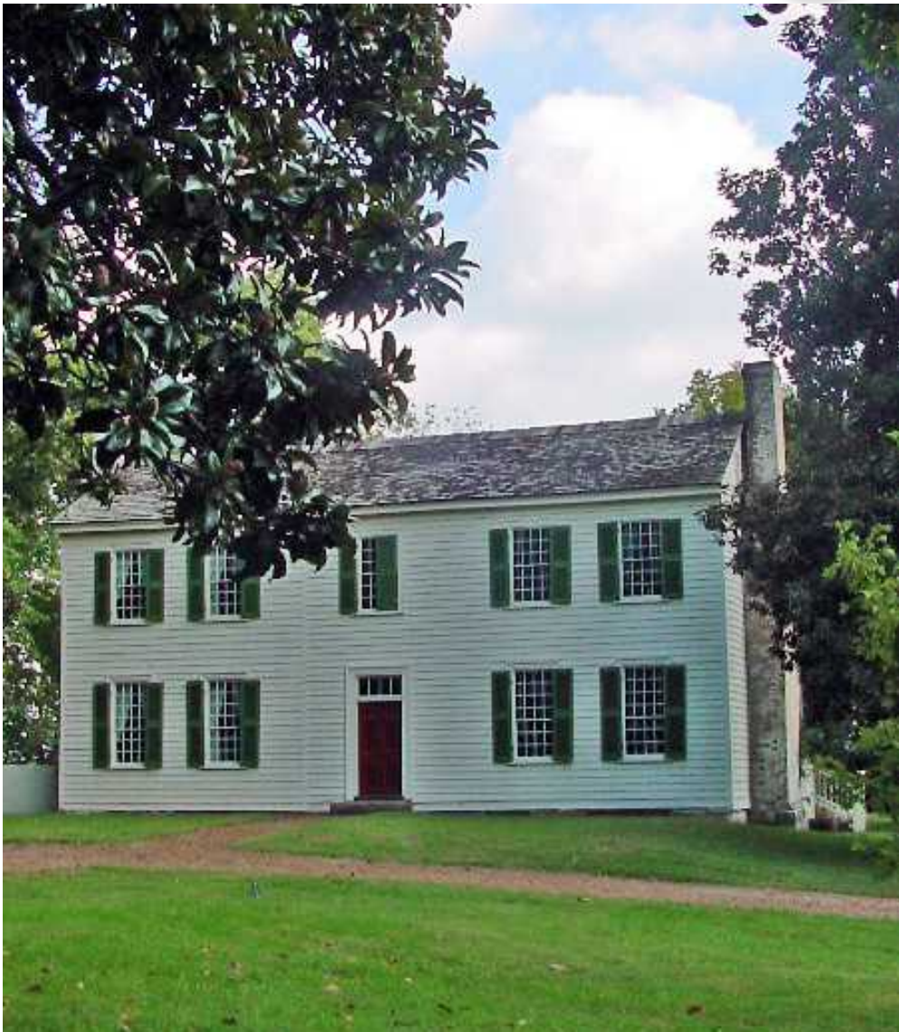
Traveller’s Rest, 1799 This house built of beaded weather boarding has undergone many changes since its early days dating back to the federalist period.
