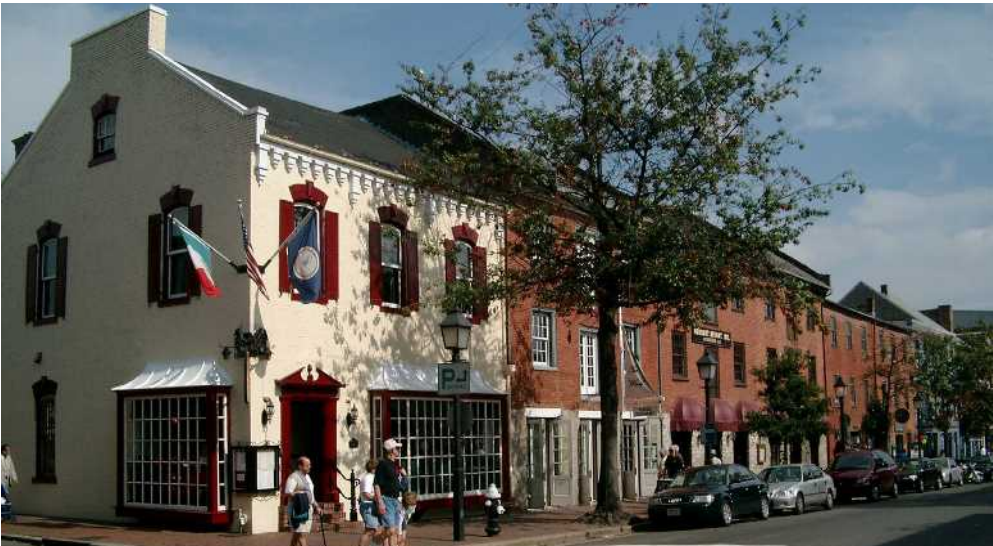
King Street, Alexandria, VA. The entry of the nearest building is to one side of the facade, as the it is below 25 feet.
