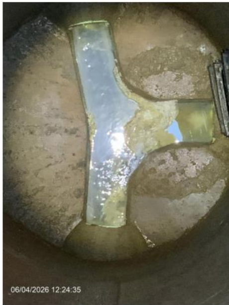
Sewer Manholes 06/04/2026 34532 First Downstream
