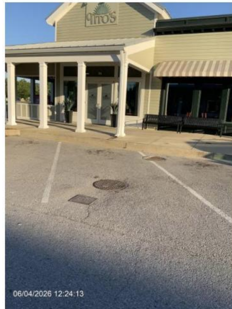
Grease Control Equipment 06/04/2026 Interceptor Location
