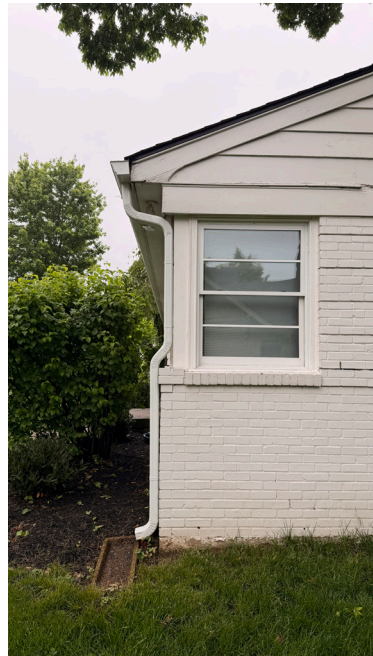
EXISTING EXTERIOR PHOTO (FOR REFERENCE)
