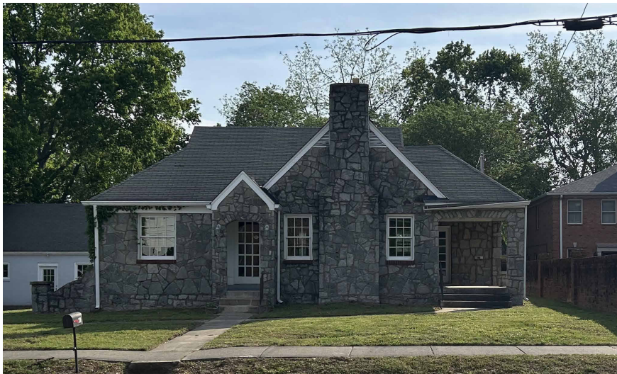
WEST STREET PHOTO
