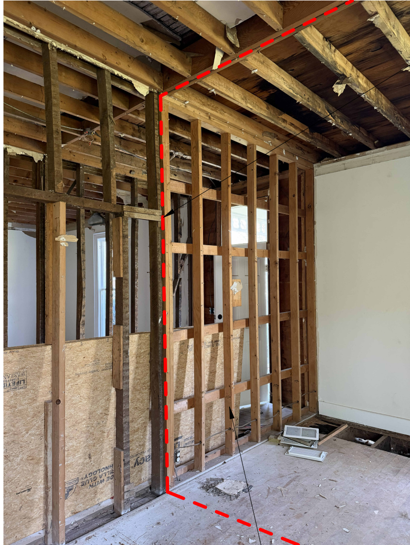
A. STUDS AND SHEATHING FROM LATER IN THE 20TH CENTURY.
