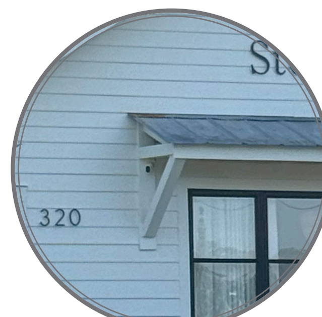
ENTRY DOOR FIBER CEMENT BRACKET PROFILE
