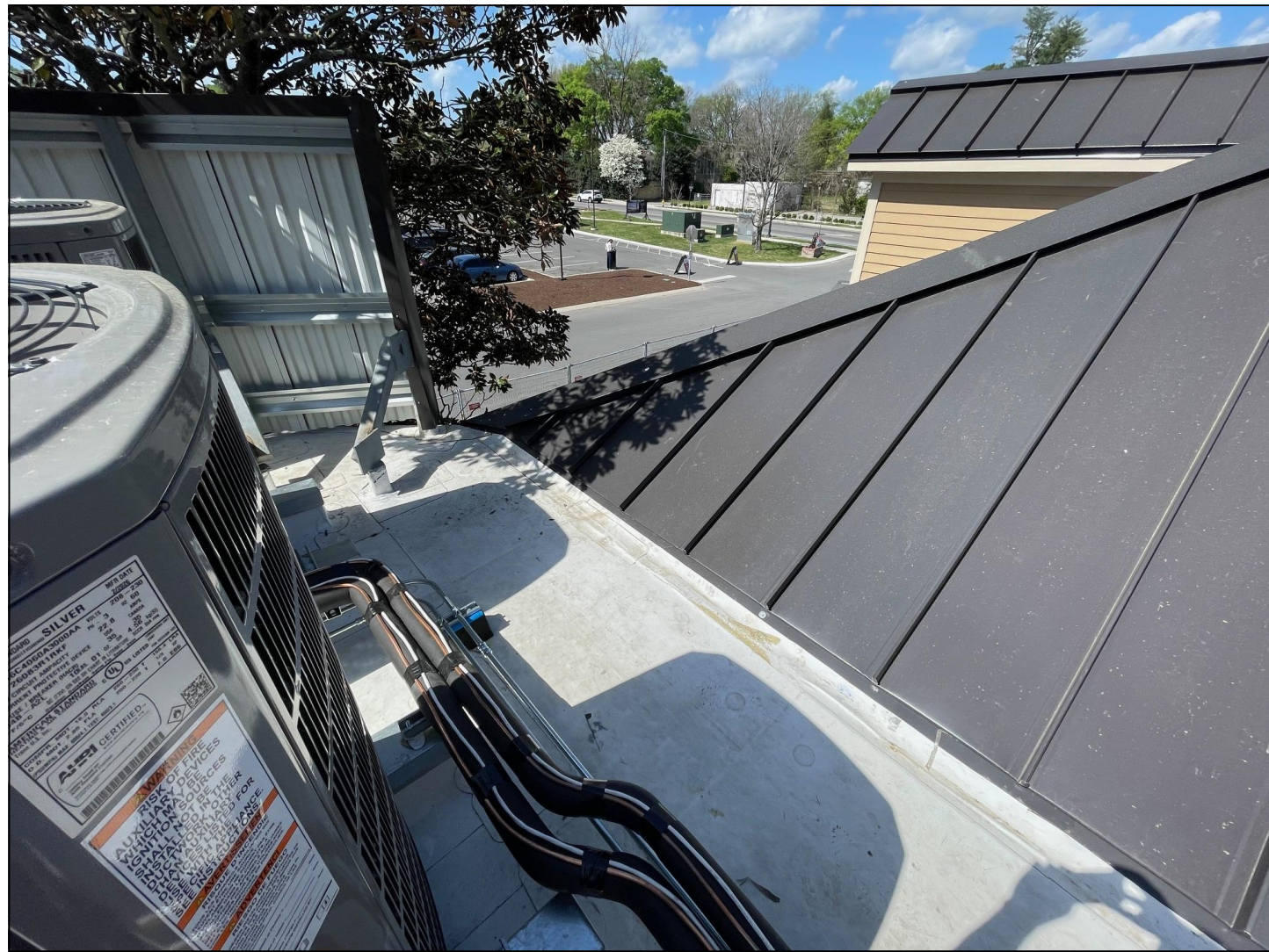
EXISTING CONDITION VIEWED FROM THE MECHANICAL PLATFORM .
