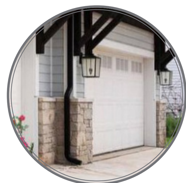
APPARATUS BAY DOOR FIBER CEMENT TRIM 1" X 11.25" HEAD TRIM, 1" X 5.5" JAMB TRIM
