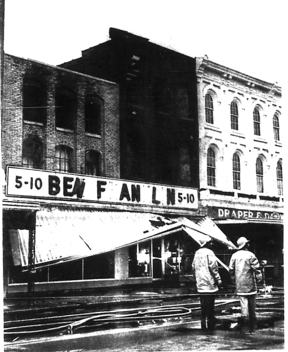
Firemen continued a watch at the Ben Franklin Store up into the morning Saturday to be sure the blaze that gutted the building and destroyed its contents was completely out. The block of Main Street just west of the Public Square was closed much of the day. After firemen left a large crane was brought in to remove the awning and the roofing that had collapsed inside the building.
