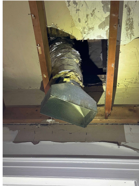
C. WHILE DIFFICULT TO SEE IN PHOTOGRAPHS, THE FRONT GABLE HAS BEEN REPAIRED WITH NEW STUDS AND PLYWOOD SHEATHING BENEATH THE VINYL SIDING. ALSO VISIBLE FROM THIS HOLE SHOWS THE ROOF UNDERLAYMENT TO BE PLYWOOD AND NOT OF HISTORIC MATERIALS.
