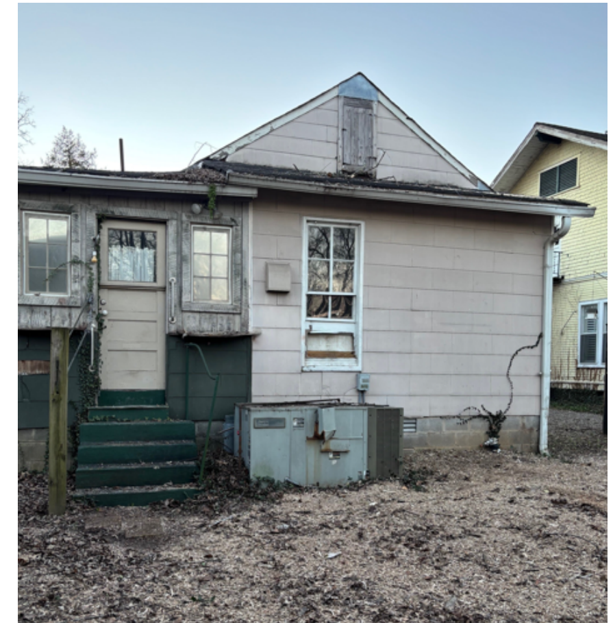
EXISTING CONDITIONS AT REAR OF HOUSE AND 42\"/>
