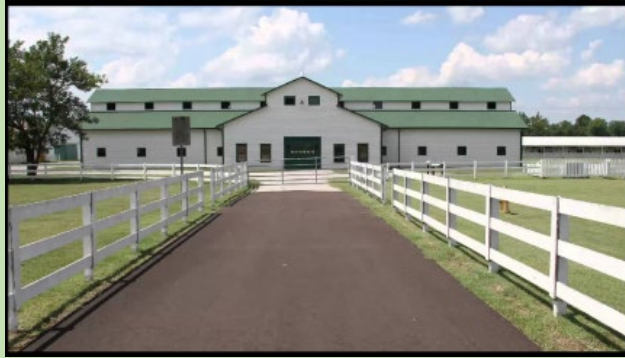
Main Barn/Events @ HF Personnel:
