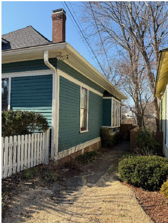
Side Elevation Figure 3 – Side view of the structure.
