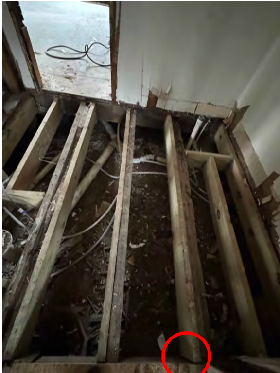
C. NEW FRAMING AT INTERIOR LOCATIONS. SISTERD ALONG JOISTS WITH GAPS AND NO FASTENERS.
