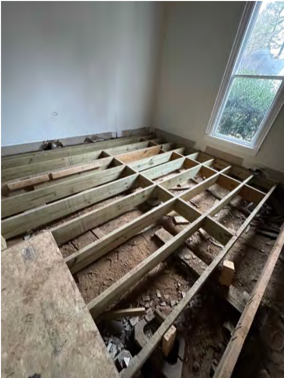
A. NEW FRAMING AT LOCATIONS THROUGHOUT. JOISTS ARE NOT LEVEL AND THERE IS DEFLECTION AMONG JOIST. NO HANGERS OR PROPER FASTENERS.
