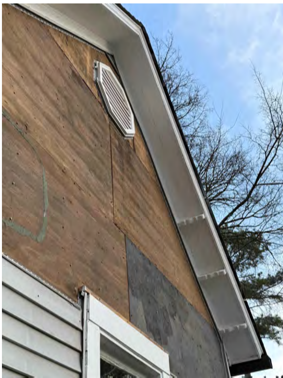
B. EXTERIOR FRAMING BOWS
