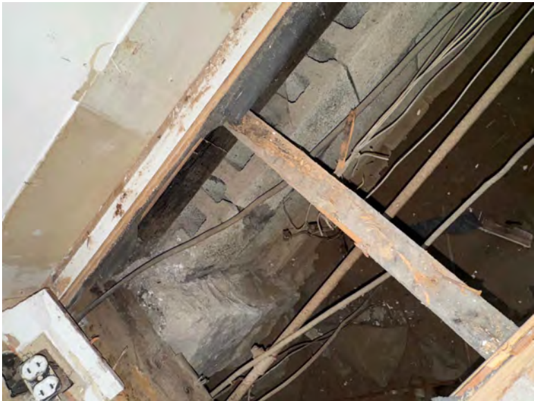
F. CMU FOUNDATION. NOT GROUTED. BEARING ON DIRT.
