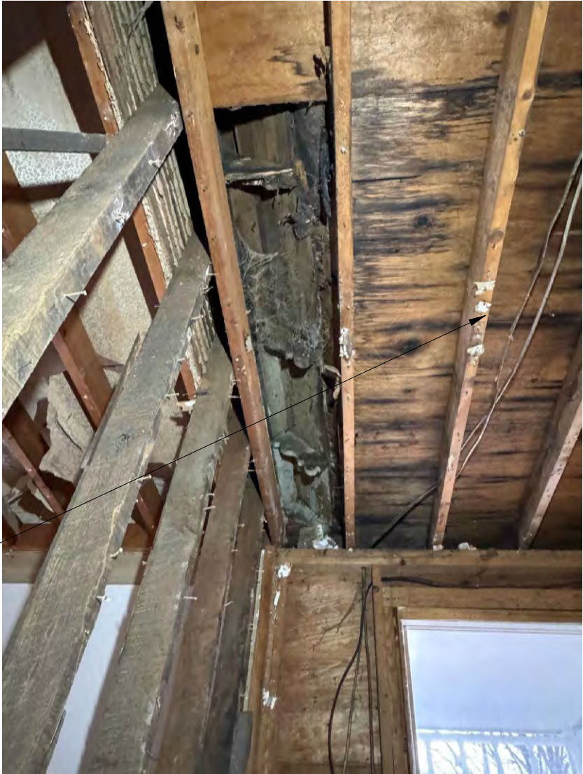
B. EXPOSED RAFTER TAILS FROM FRONT GABLE SEEN INSIDE OF FRONT ROOM CEILING. THIS INDICATES THAT THE PORCH ROOF SLOPE WOULD HAVE BEEN LOWER THAN THESE RAFTER TAILS AND THESE WOULD HAVE BEEN SEEN FROM THE FRONT OF THE HOUSE.
