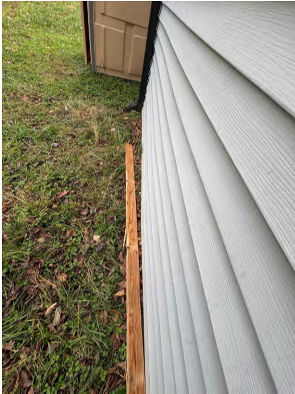
B. EXTERIOR FRAMING BOWS
