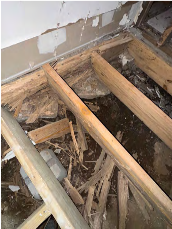
B. HISTORIC RIM BOARD IS DETERIORATED BY TERMITE DAMAGE.
