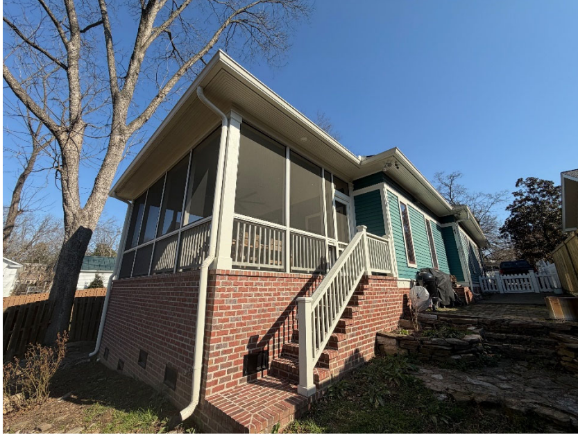
Rear Elevation Figure 2 – Rear view of the structure.
