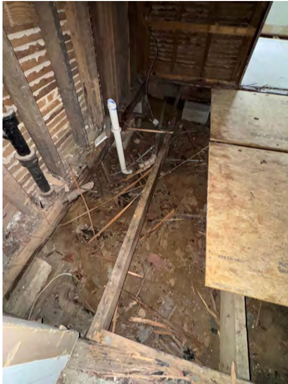
D. HISTORIC JOISTS HAVE COLLAPSED INTO CRAWL SPACE DUE TO TERMITE DAMAGE.
