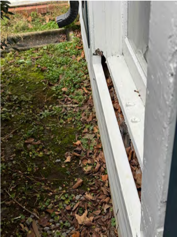
D. THE SILL IS MISSING FROM THE FRONT WINDOW. THE WALL STUDS AND FOUNDATION IS VISIBLE THROUGH THIS HOLE.
