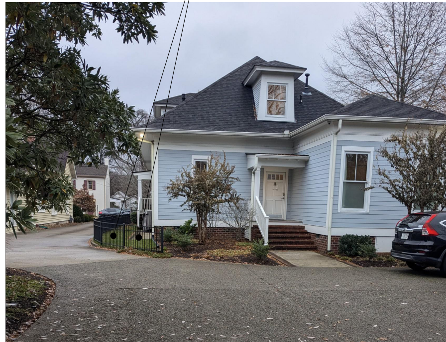
REAR ELEVATION, REAR PARKING, AND SHARED DRIVEWAY
