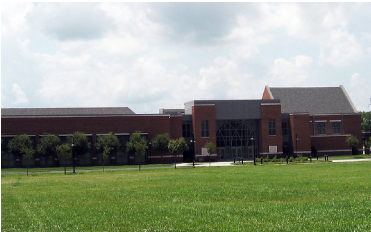
New campus for the Franklin First United Methodist | Image of the new building for the Franklin First United Methodist Church, located at 120 Aldersgate Way.
