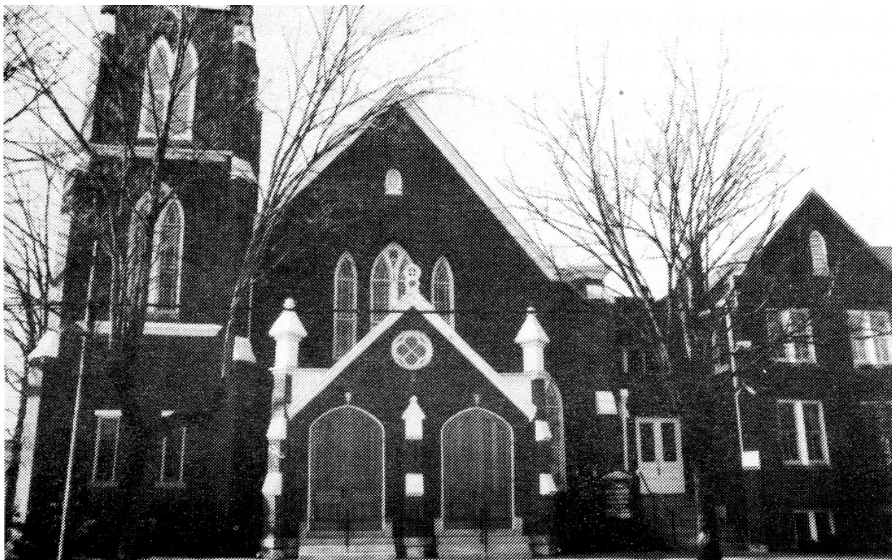
Franklin First United Methodist Church | First Franklin Methodist Church.
