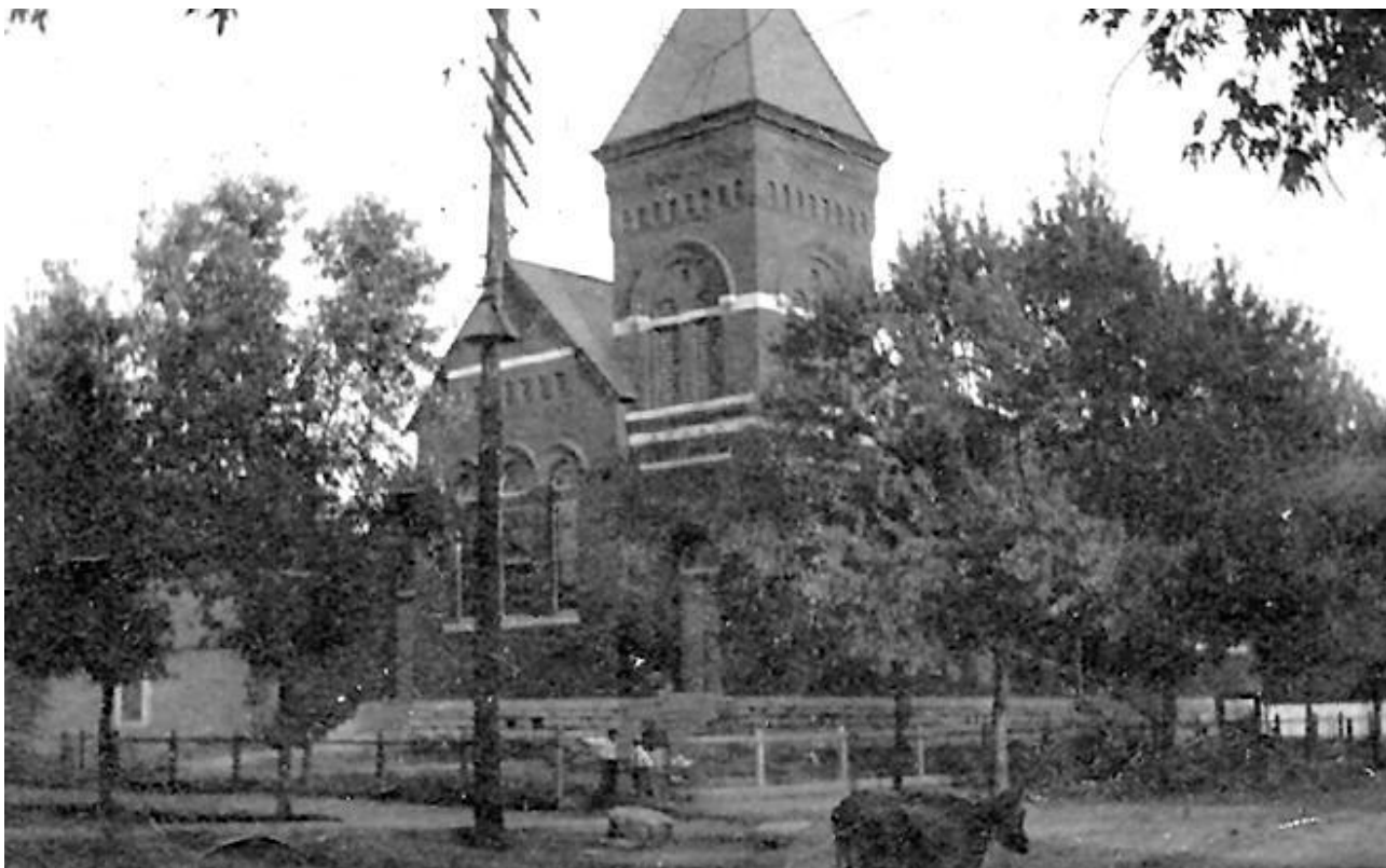
Franklin Presbyterian Church | Image of Franklin Old Presbyterian Church, ca. 1900.
