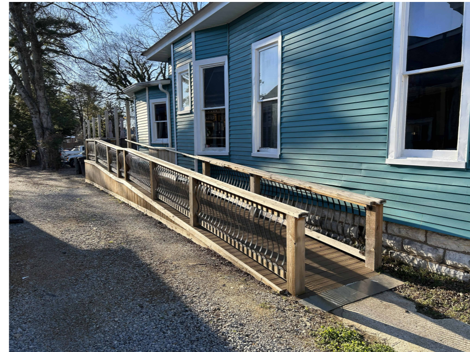
SOUTHEAST EXISTING PHOTO
