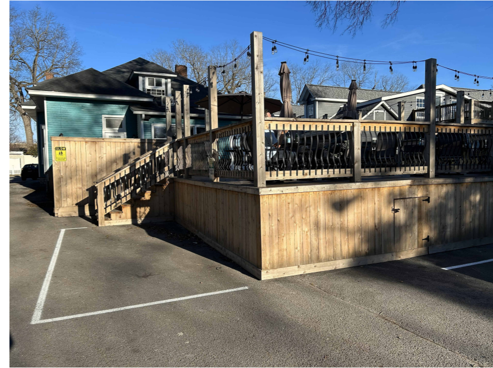
NORTHWEST EXISTING PHOTO
