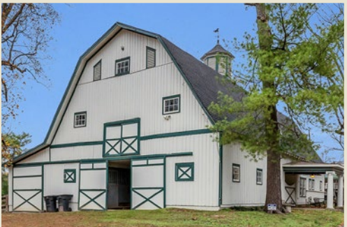
RIVERVIEW HOUSE BARN
