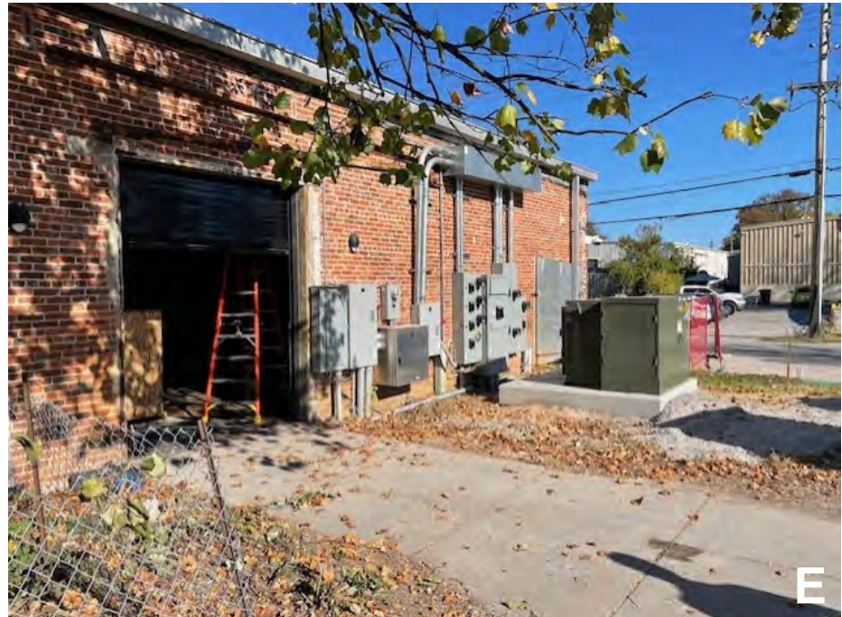
ALL EXISTING DOORS AT THE BACK OF BUILDING 5 (ADJACENT TO NEW PARKING GARAGE) TO BE UPDATED TO COMPLY WITH A 2-HR WALL RATING. REPLACED DOORS WILL BE SIMILAR IN APPEARANCE TO EXISTING.
