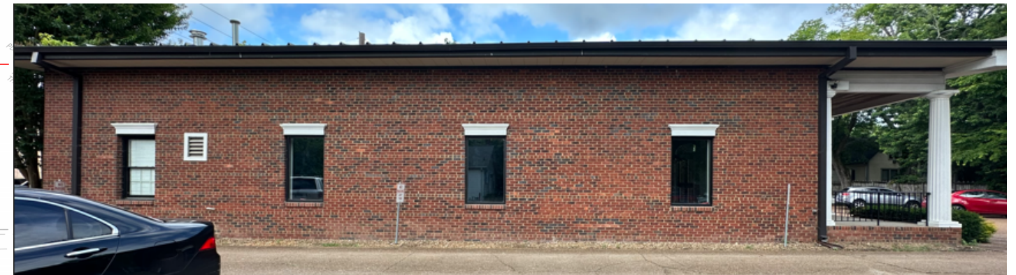
VIEW OF NON-CONTRIBUTING COMPONENT FROM THE NORTH
