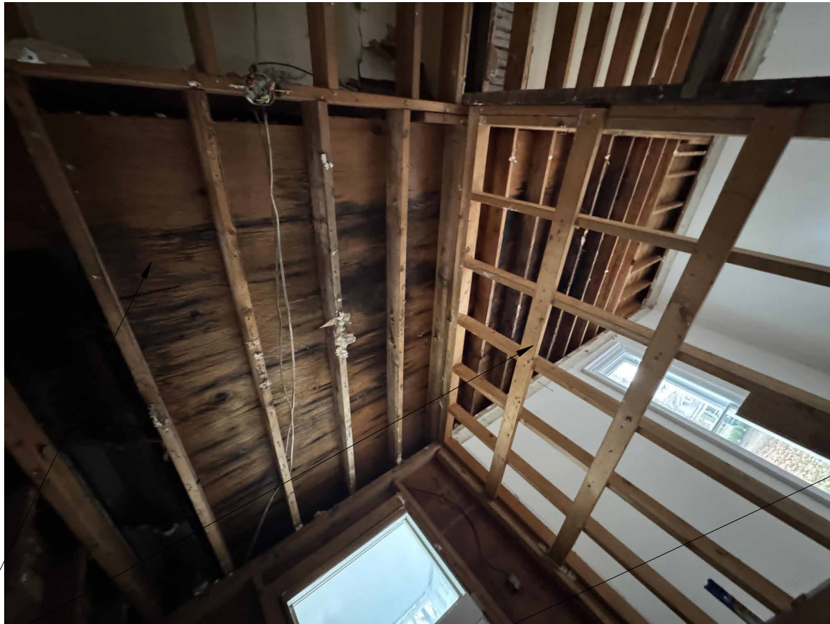
(A) STUDS AND SHEATHING FROM LATER IN THE 20TH CENTURY.
