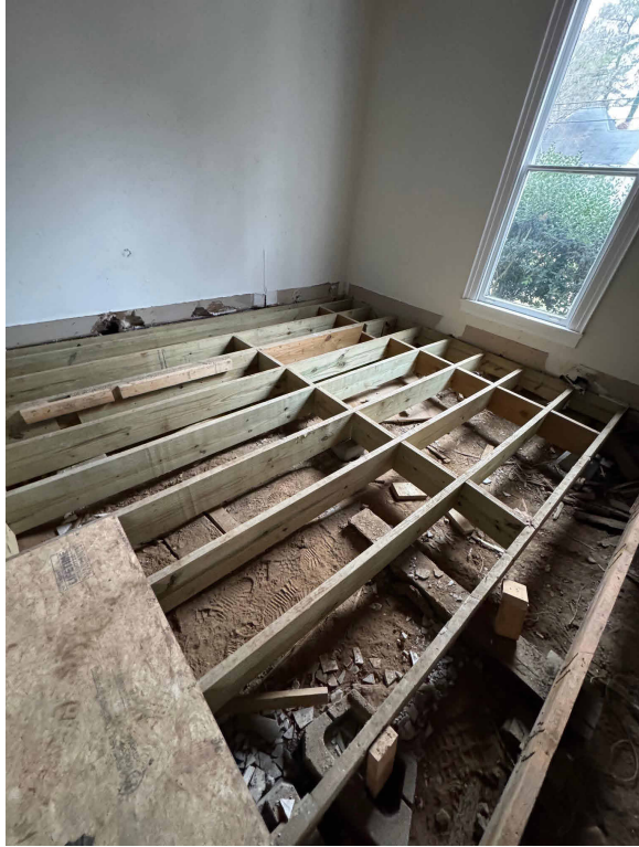
(A) NEW FLOOR FRAMING AT LOCATIONS THROUGHOUT. JOISTS ARE NOT LEVEL AND THERE IS DEFLECTION ACROSS JOIST. NO HANGERS OR PROPER FASTENERS OR CONSISTENT CONNECTION TO EXTERIOR WALLS
