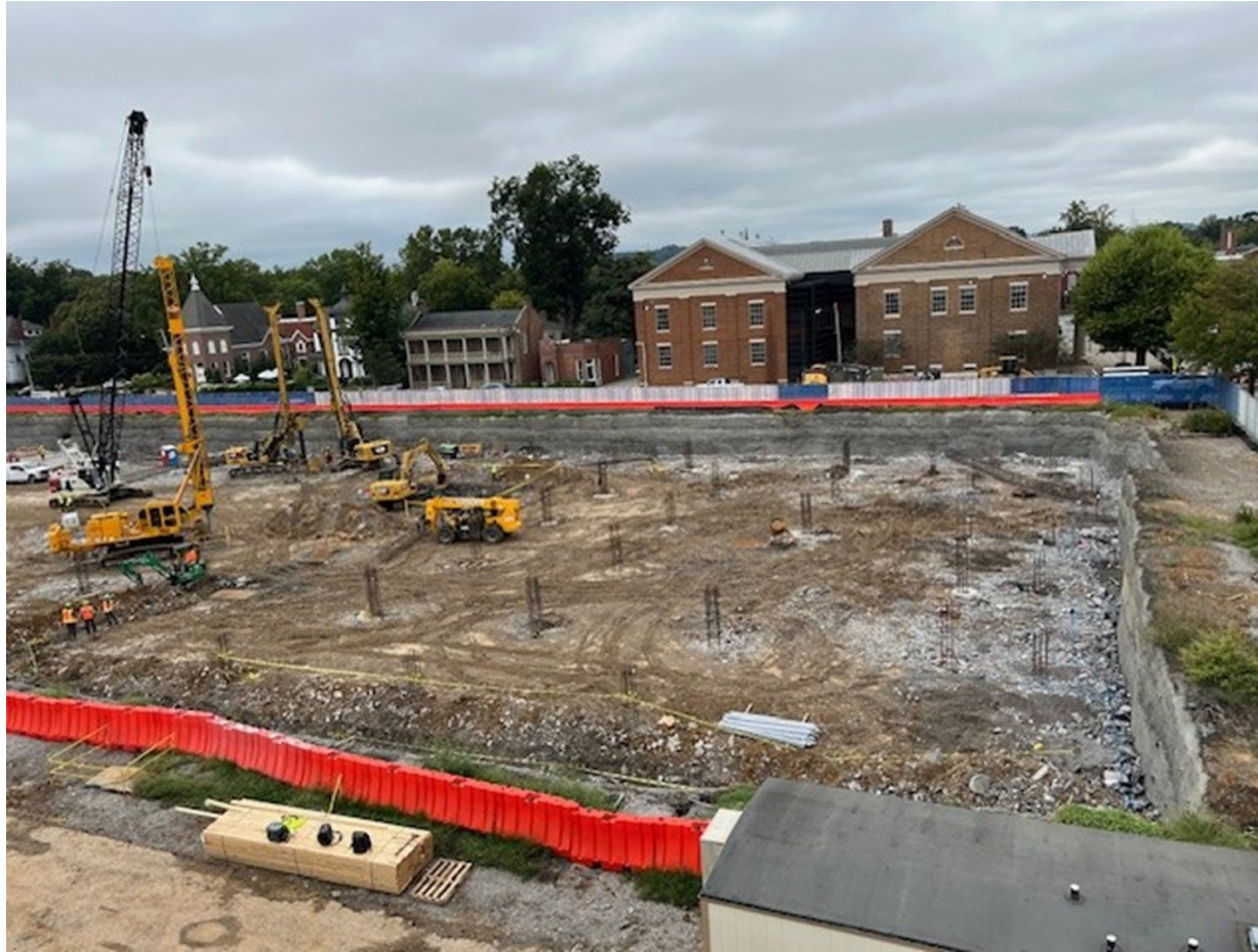
AREA A Sub-Surface Piers October 2025
