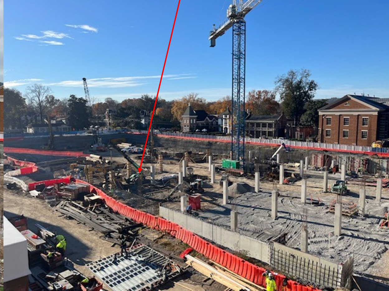
AREA B Columns and Walls November 2025
