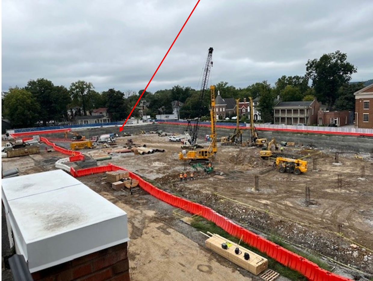
AREA B Sub-Surface Piers October 2025
