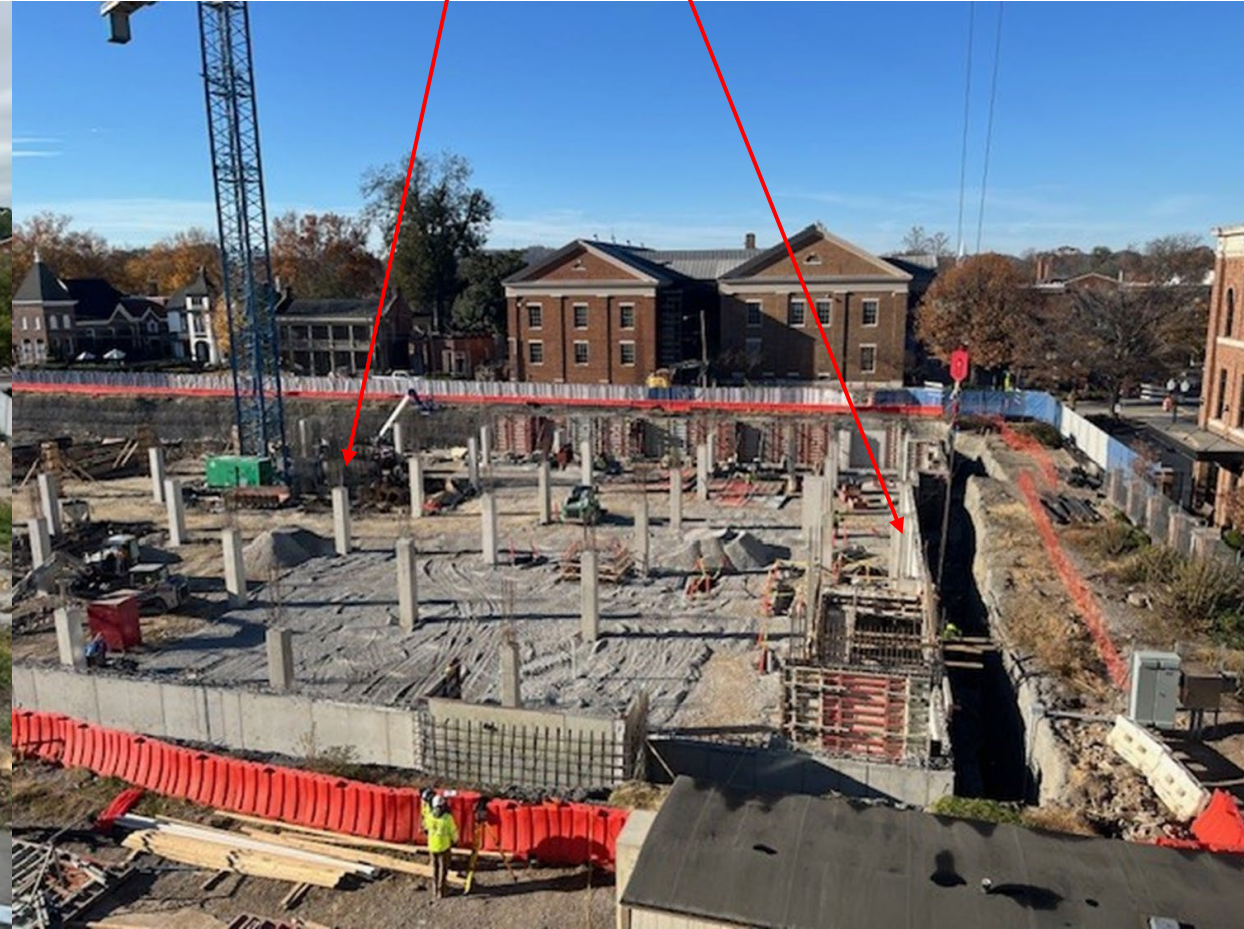
AREA A Columns and Walls November 2025
