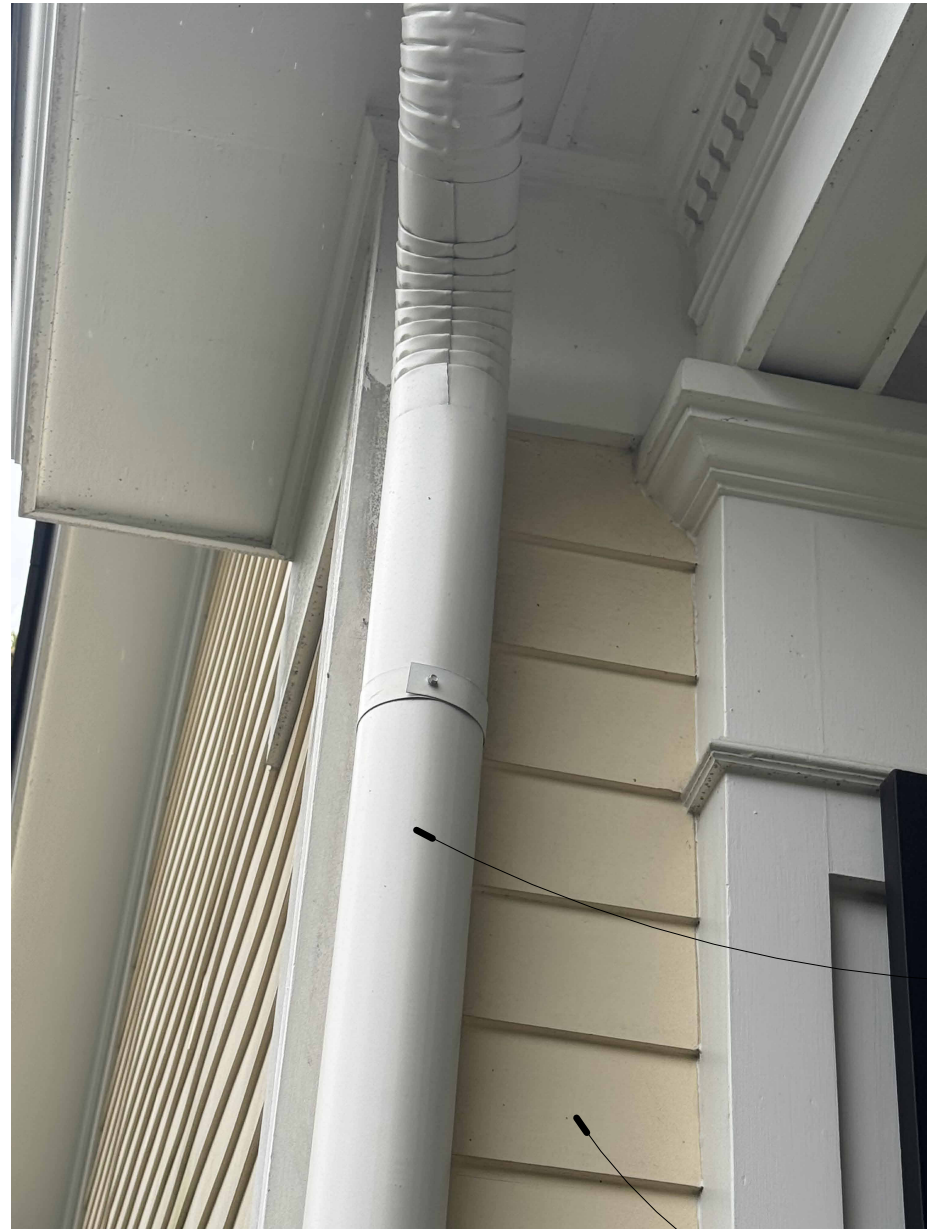
EXISTING WHITE PREFINISHED DOWNSPOUT
