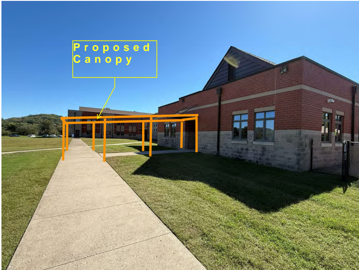
Photo #6. North Elevation Mustard Looking East
