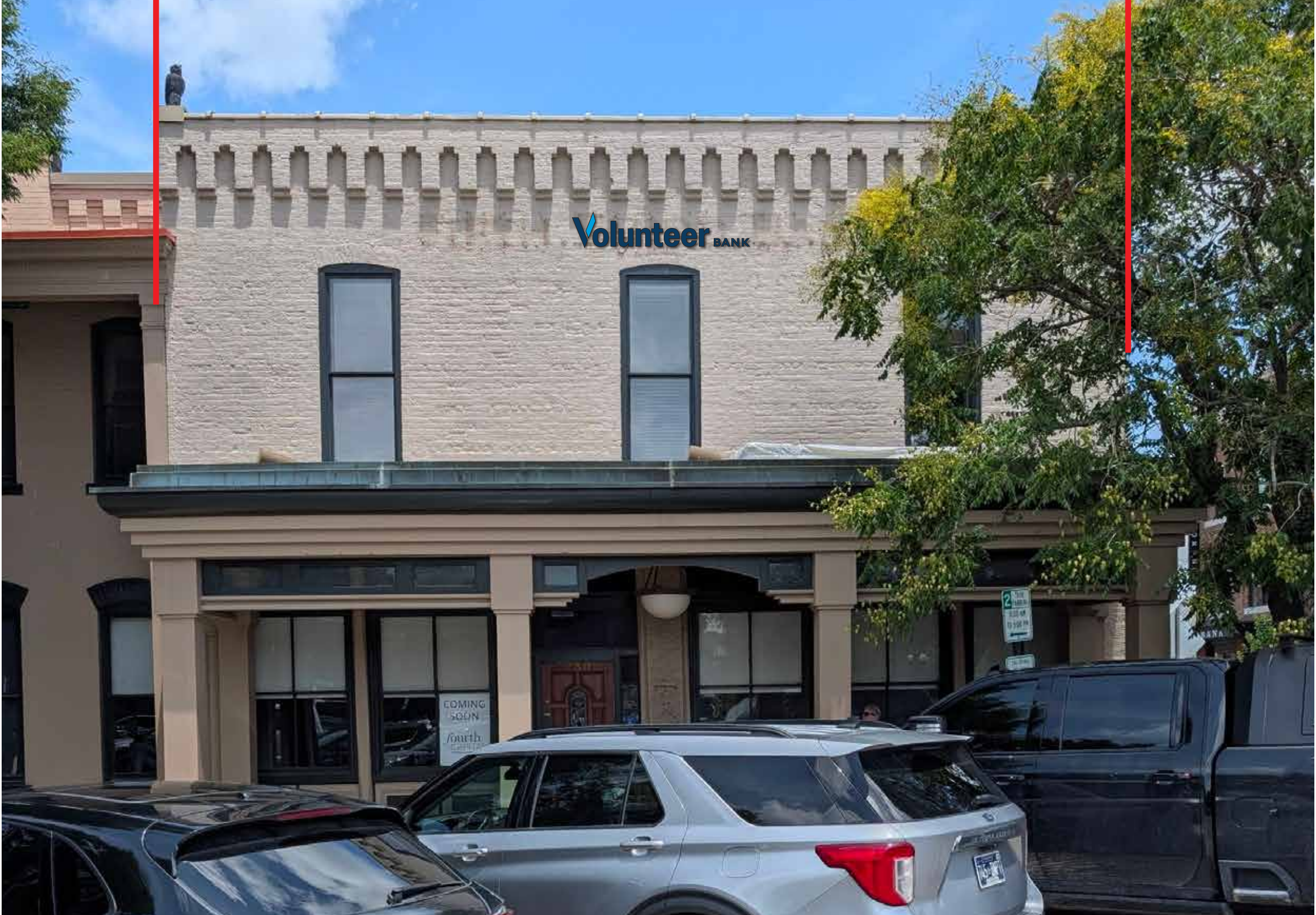
16" HEIGHT, 1/2" THICK ALUM FLAT CUT OUT LOGO SERVICE AND FOCUS EXISTING LIGHTS
