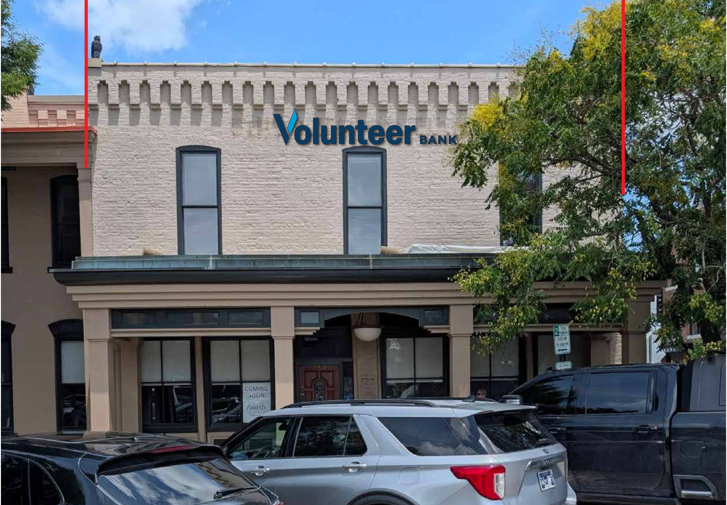
30" HEIGHT, 1/2" THICK ALUM FLAT CUT OUT LOGO SERVICE AND FOCUS EXISTING LIGHTS
