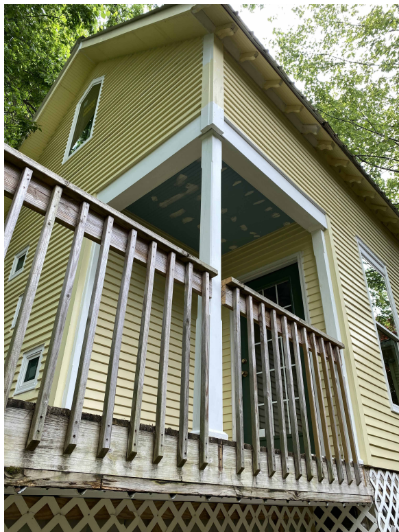
EXISTING: LEFT SIDE @ REAR
