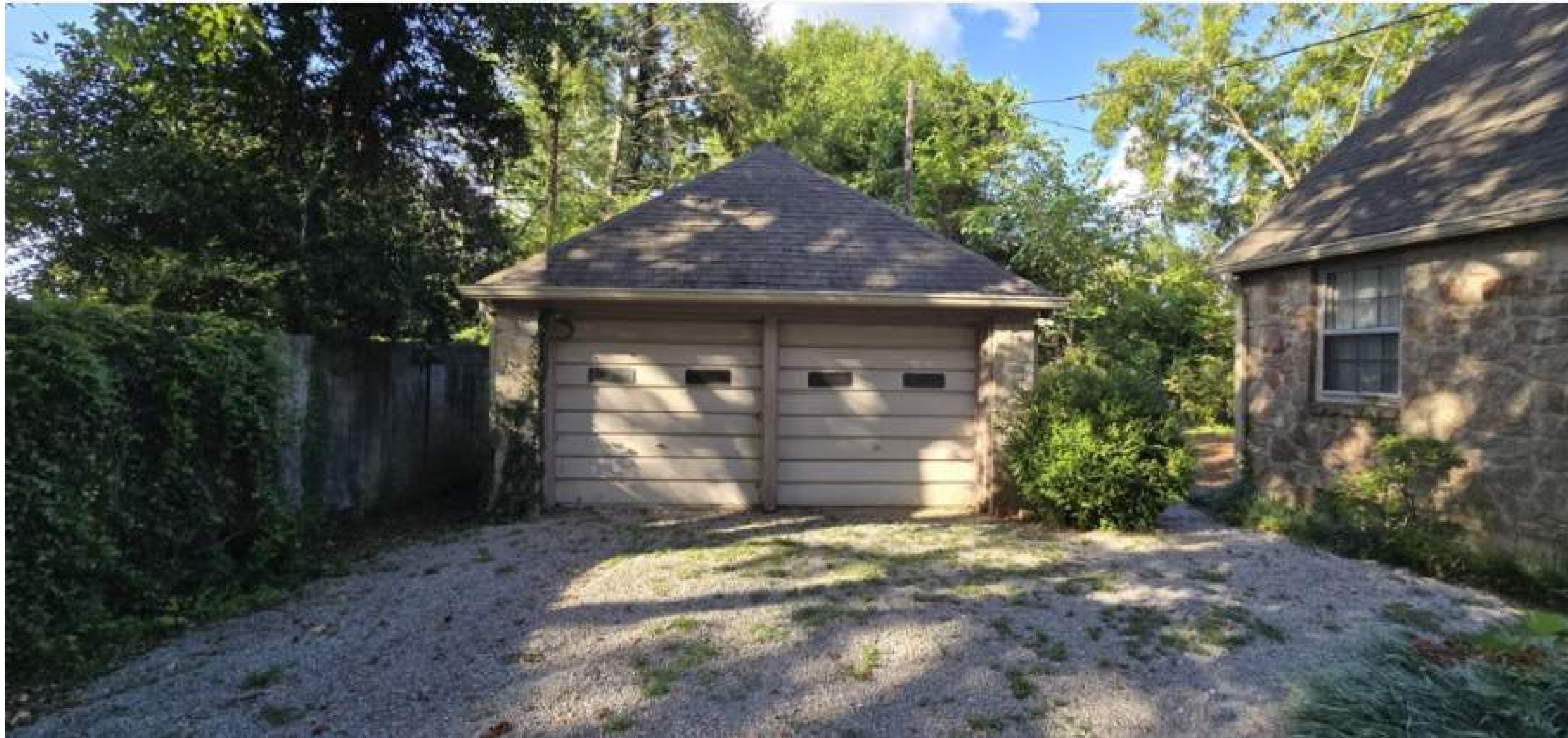
Existing Garage Winslow Road Elevation - for reference
