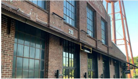
EXISTING LINEAR LIGHTS ON BUILDING 11 DIRECTLY BEHIND BUILDING 1
