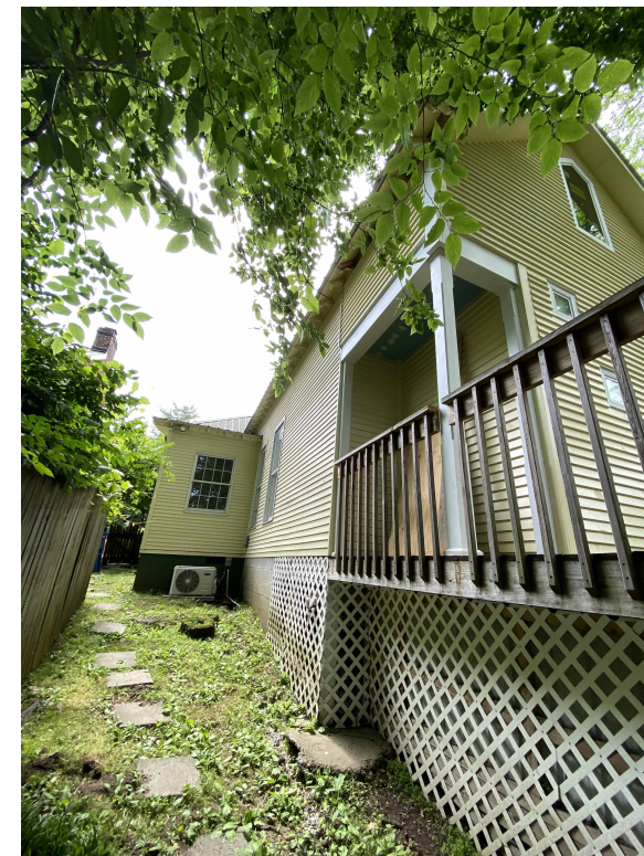
EXISTING: RIGHT SIDE @ REAR
