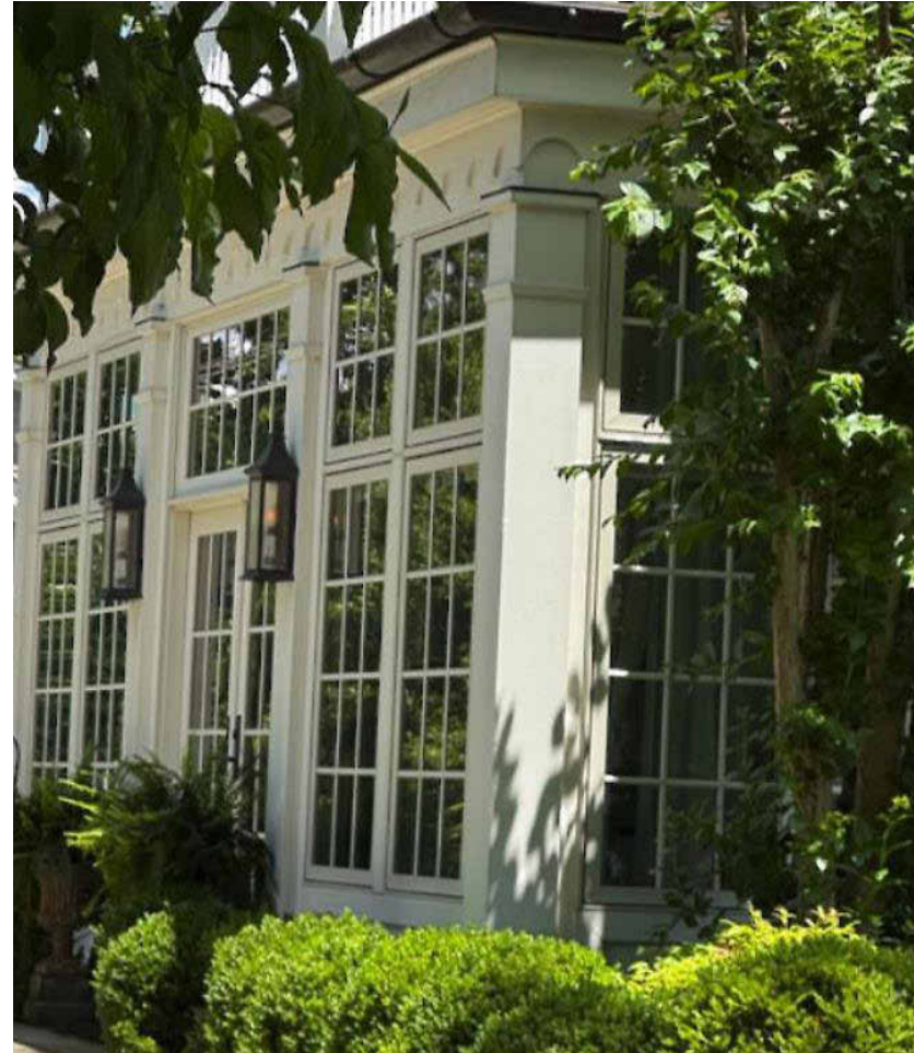
235 3RD AVE SOUTH
