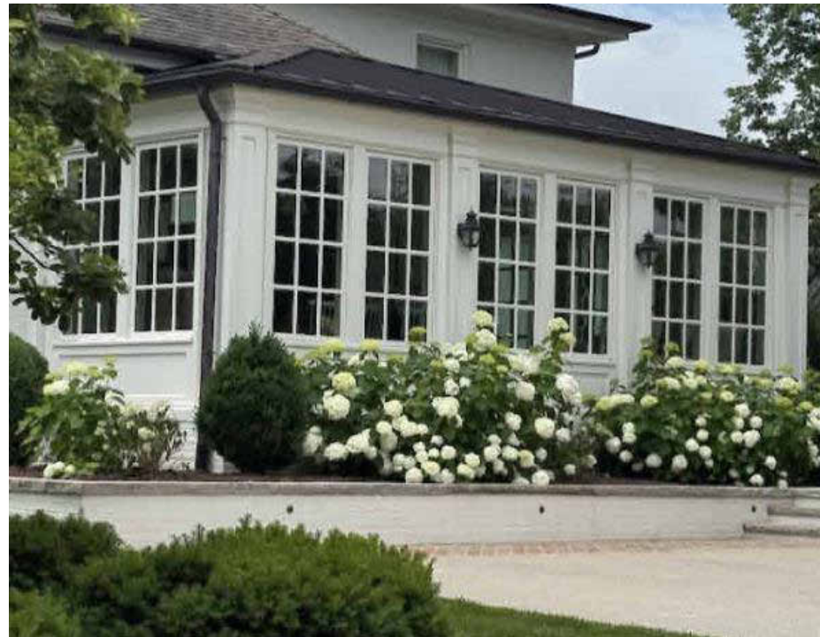
243 3RD AVE SOUTH
