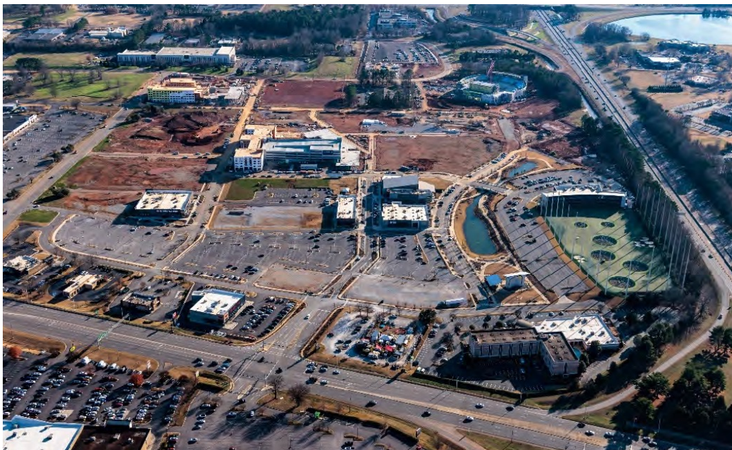
Ariel View from the North (December 14, 2021)
