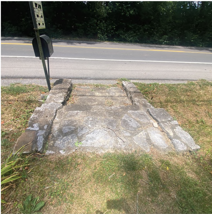
Existing stone stairs and mailbox on site
