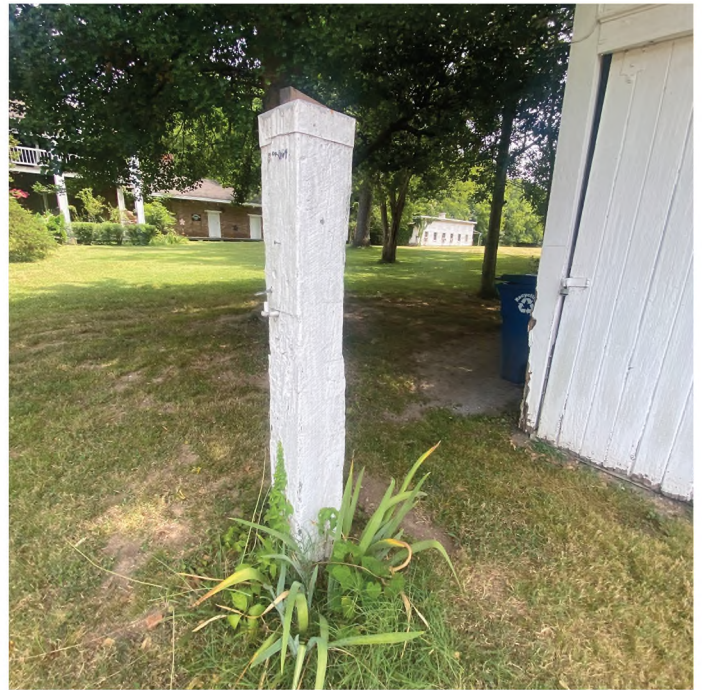
Existing springhouse on site
