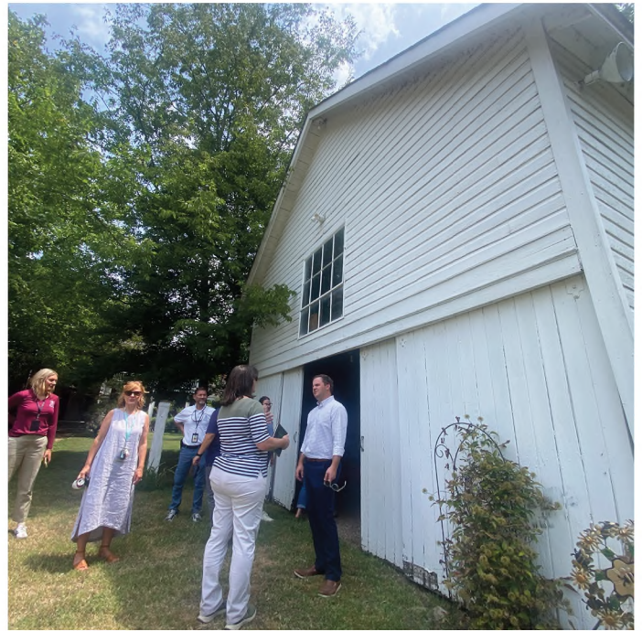
Existing structure on site
