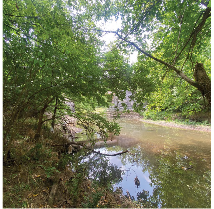
Spencer Creek and existing railroad bridge crossing
