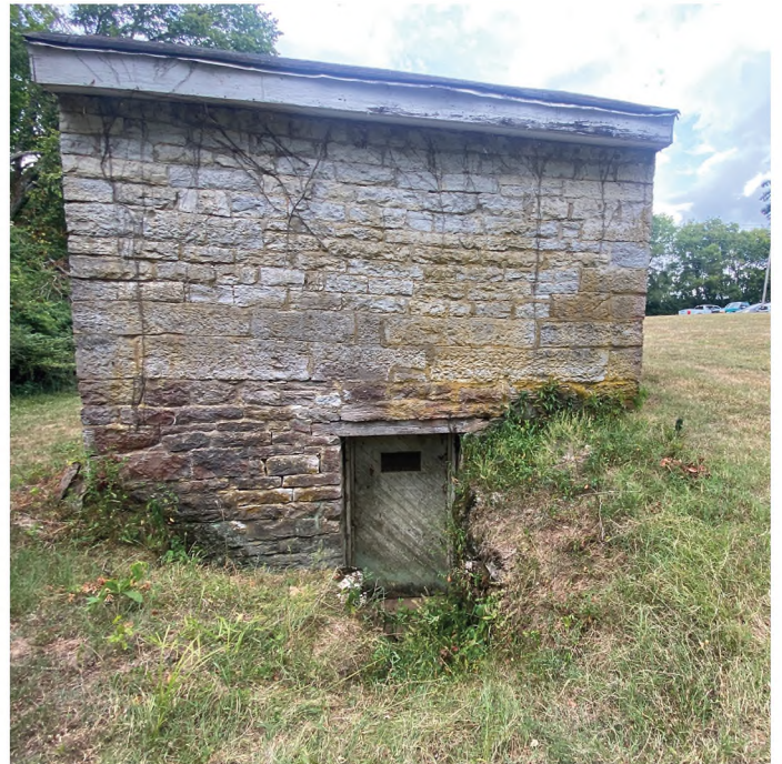
Existing structure on site
