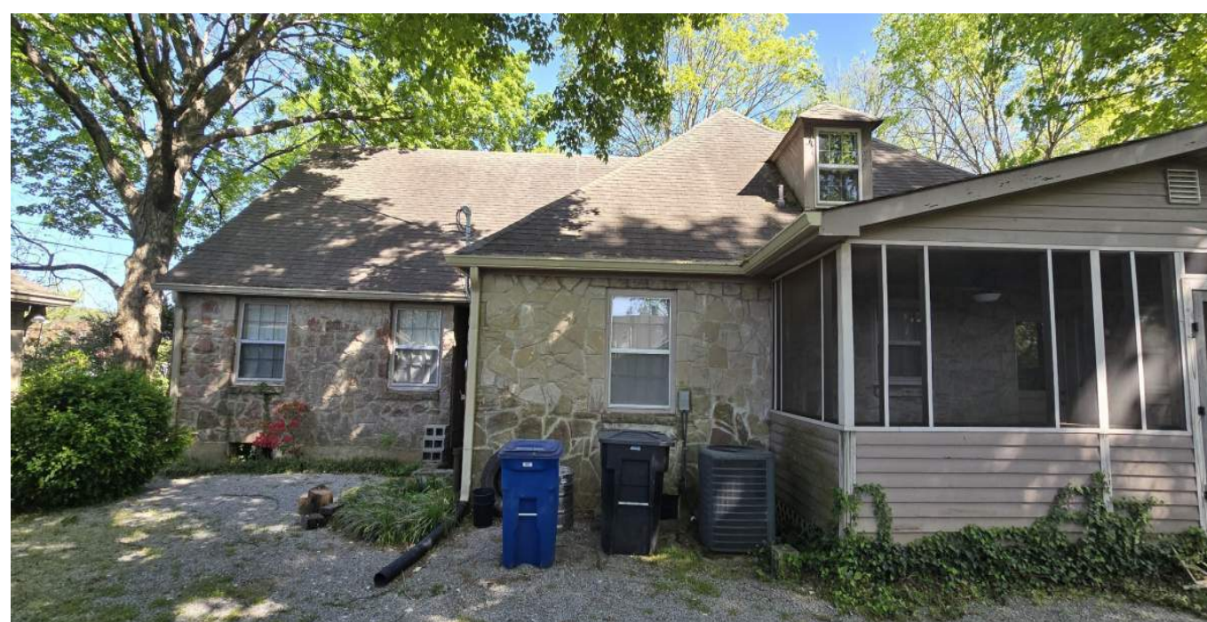
Left side elevation with utilities and open basement access
