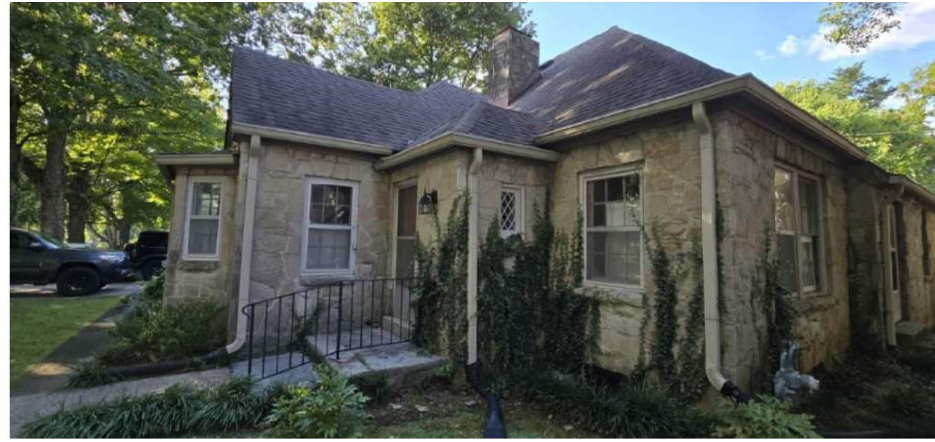
Entry detail / cornice and roof condition
