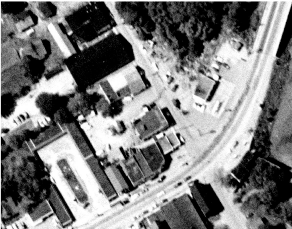
Figure 8 1958 aerial of East Main St. showing a new service station and old buildings demolished.
