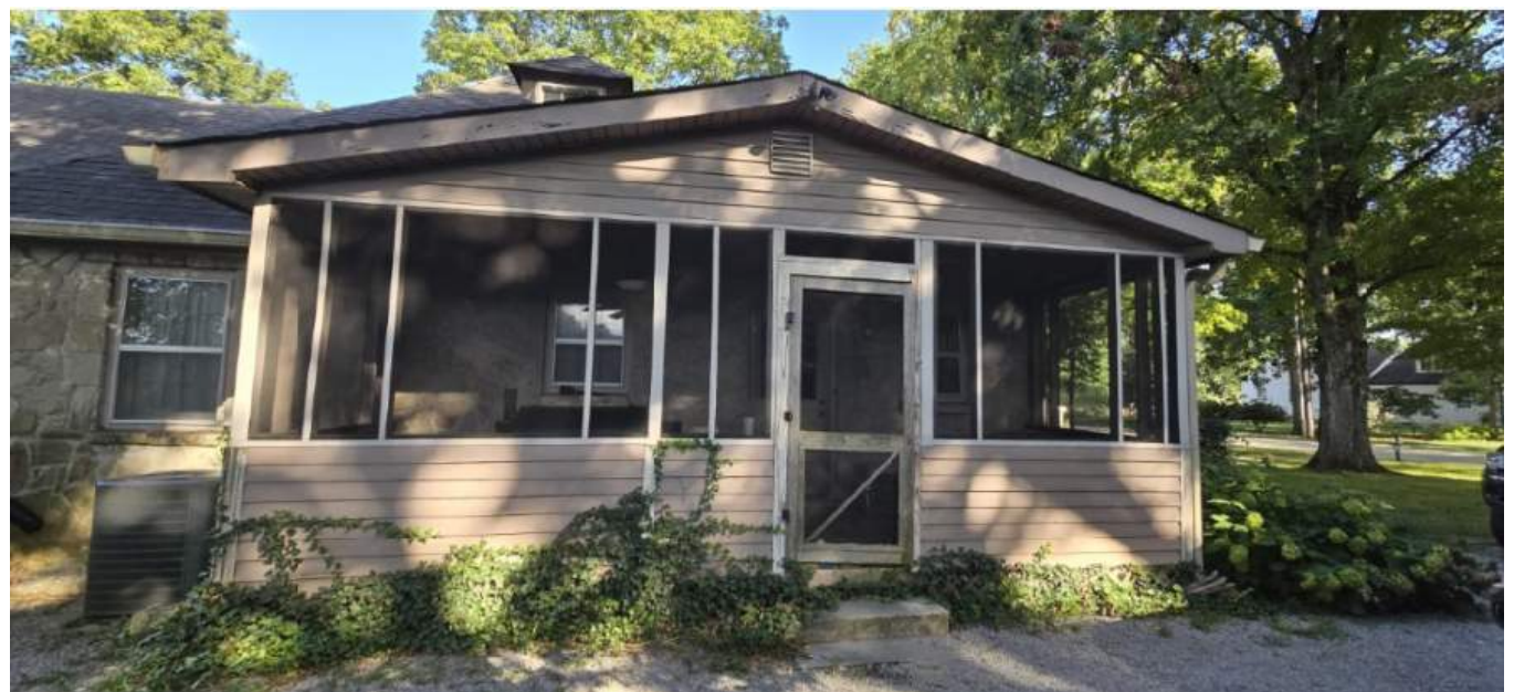
Screen addition - COA granted 2008
