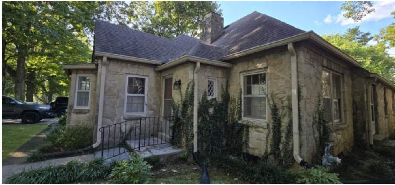
Entry detail / cornice and roof condition
