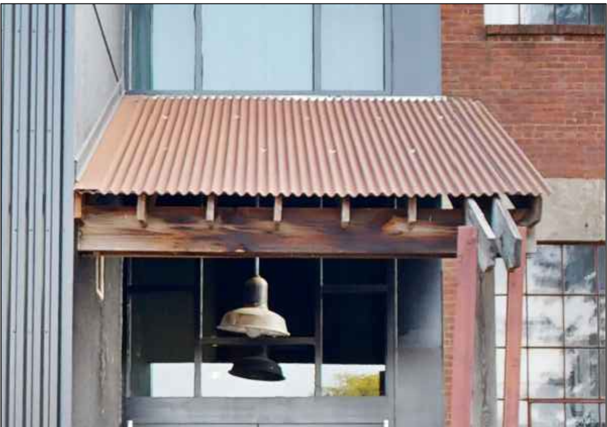
EXISTING SITE CONTEXT FOR AWNING @ REAR ENTRANCE INTO BUILDING
