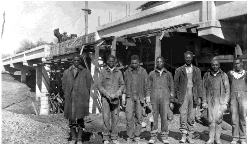
Figure 2 Franklin Road bridge workers circa 1928. Black American men represented a significant workforce of brick/stone masons and concrete workers.
