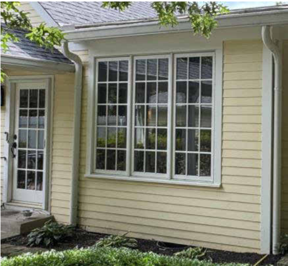
EXISTING WINDOWS AT DEN
