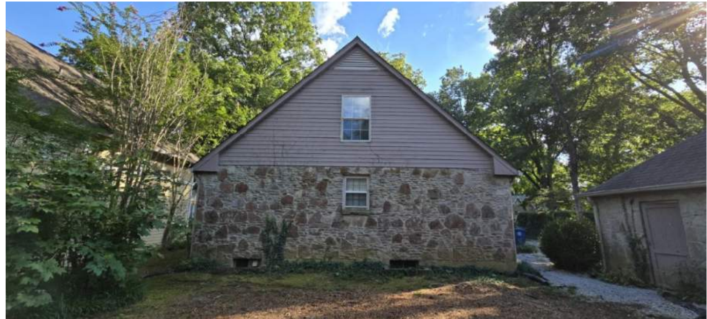
Rear elevation of 1970's addition
