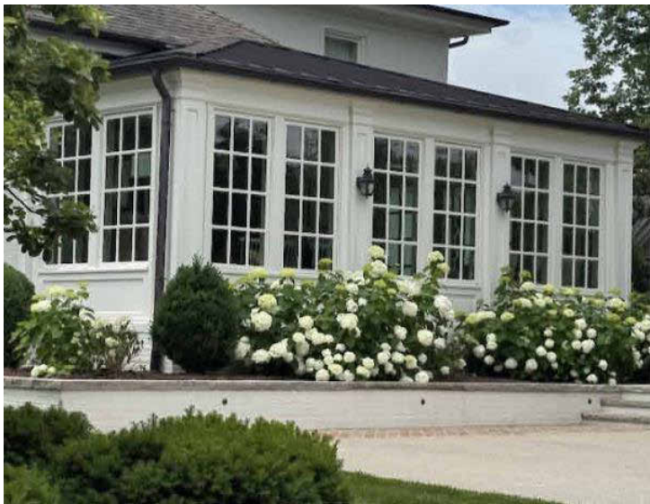
243 3RD AVE SOUTH
