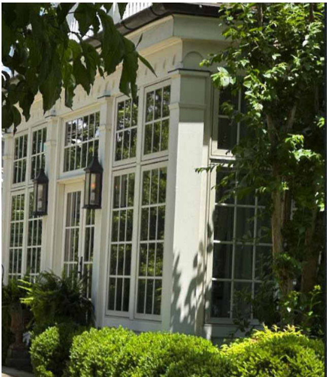
235 3RD AVE SOUTH
