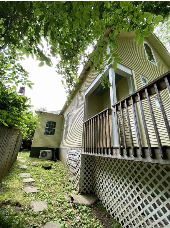
EXISTING: RIGHT SIDE @ REAR
