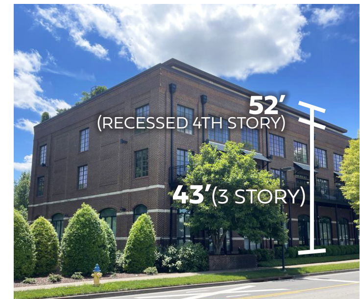
JAMISON STATION HEIGHT
