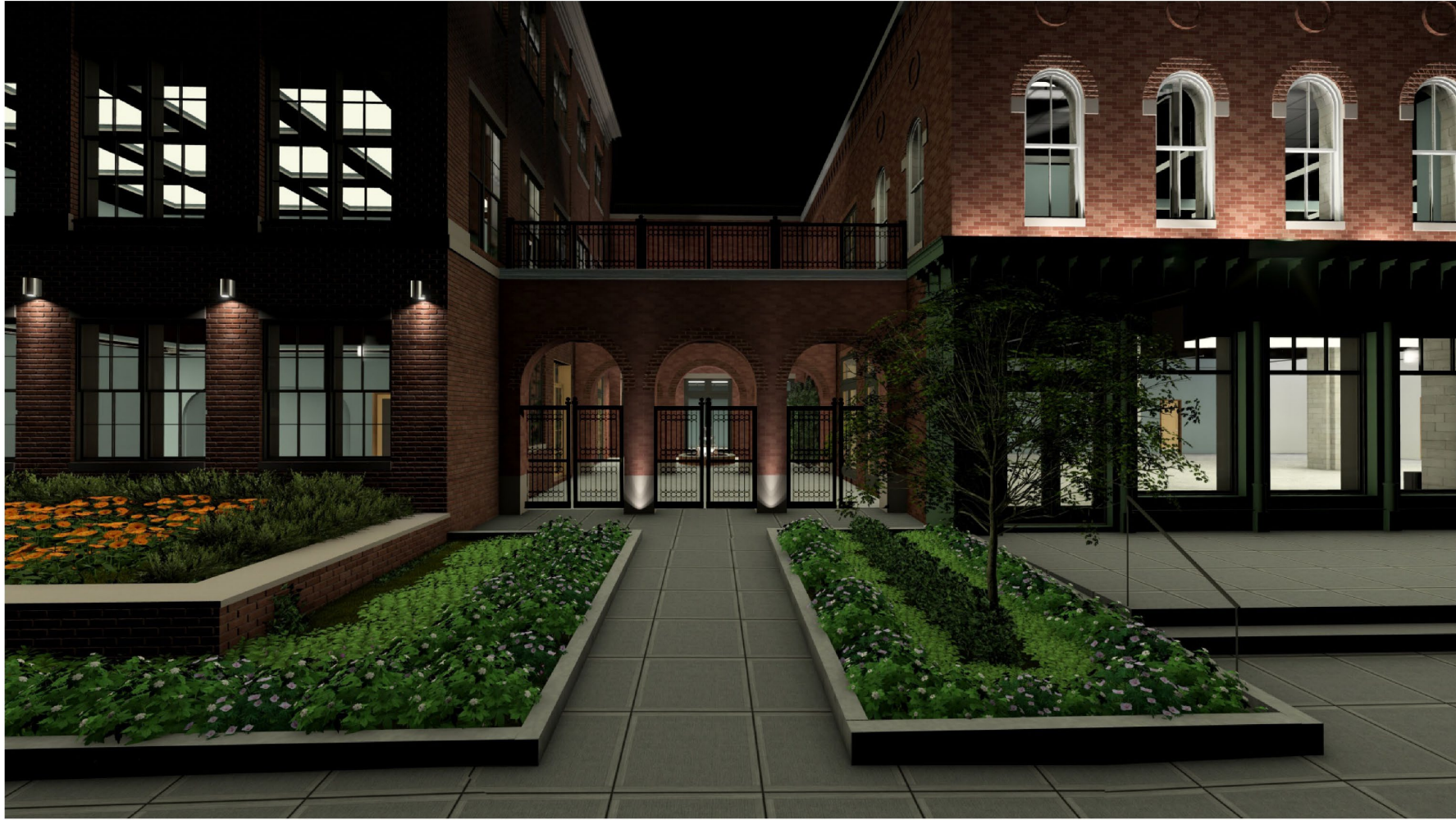
LIGHTING AT COURTYARD
