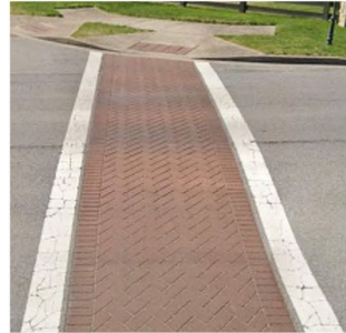
CITY OF FRANKLIN STAMPED ASPHALT CROSSWALK P-111
