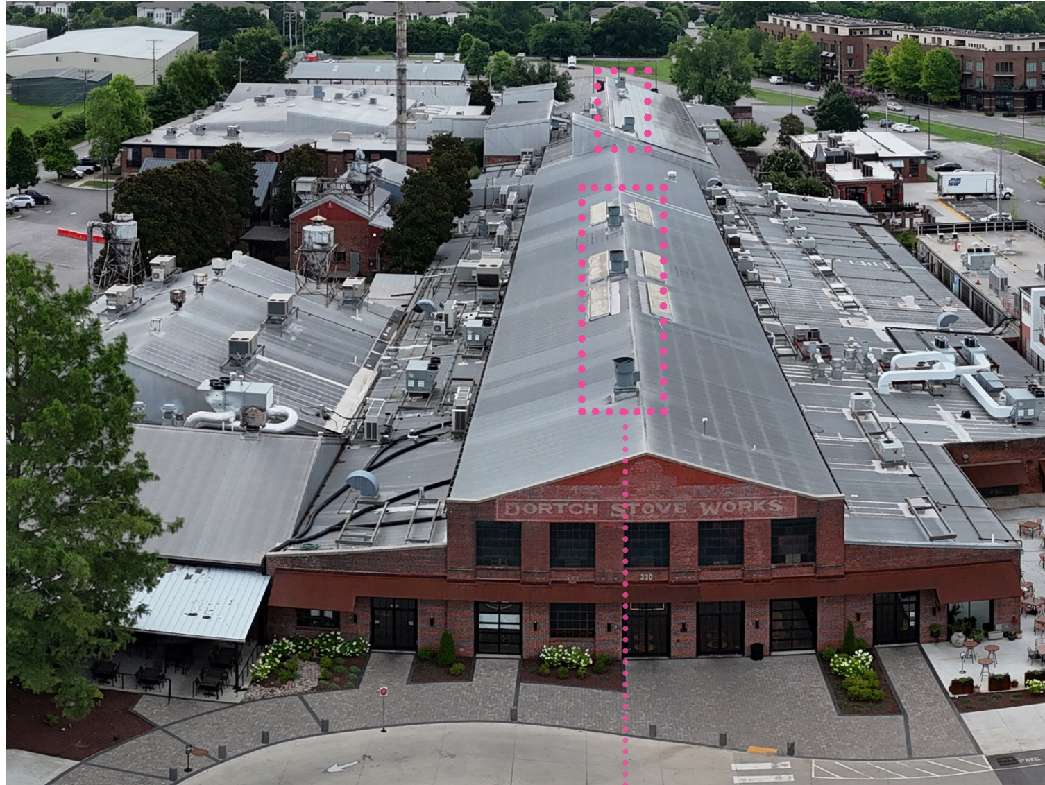
EXHAUST FAN APPEARS IN THE FACTORY ARCHITECTURAL VERNACULAR
