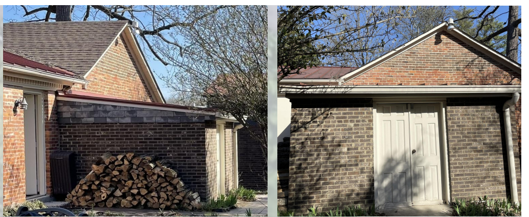
CURRENT CONDITION OF STORAGE ADDITION
