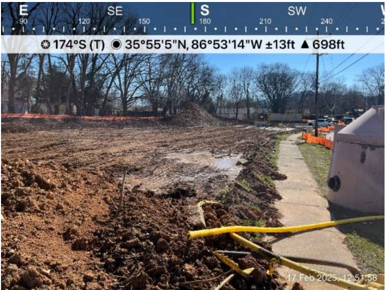
View of Shawnee site cut to subgrade, standing water
