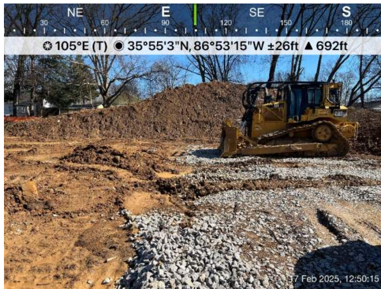
View of end of construction entrance and soil stockpile on Shawnee site
