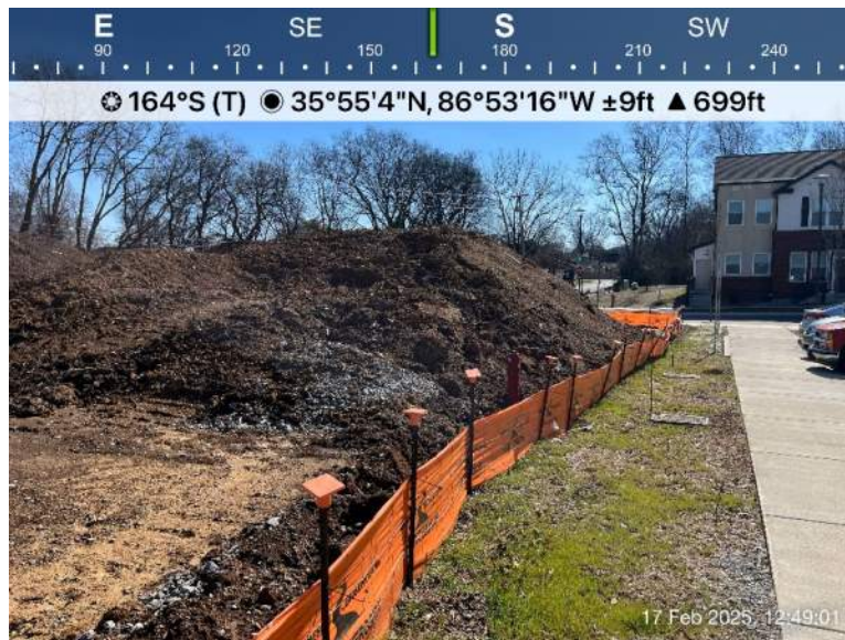
Soil stockpile on south end of Cherokee site
