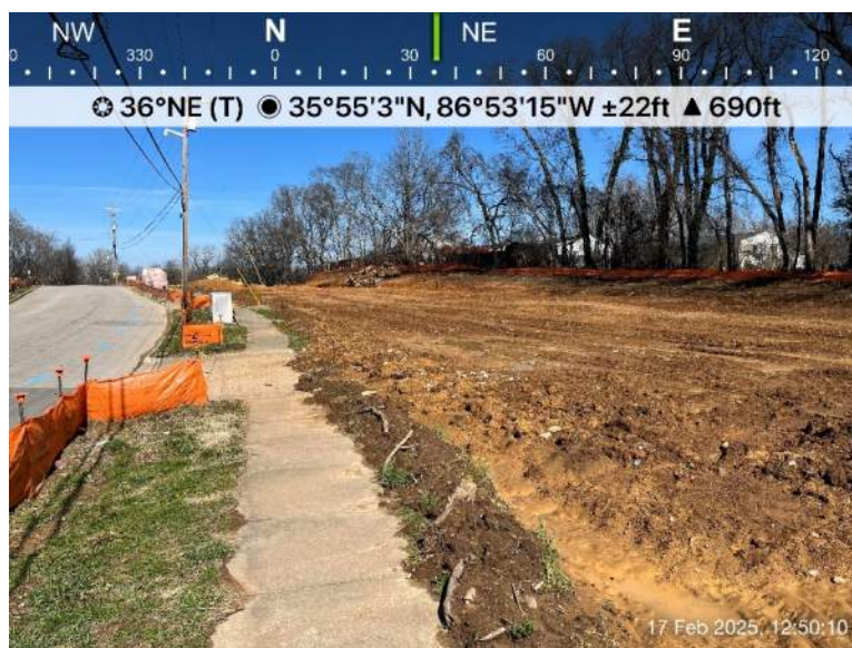
View of Shawnee site cut to subgrade
