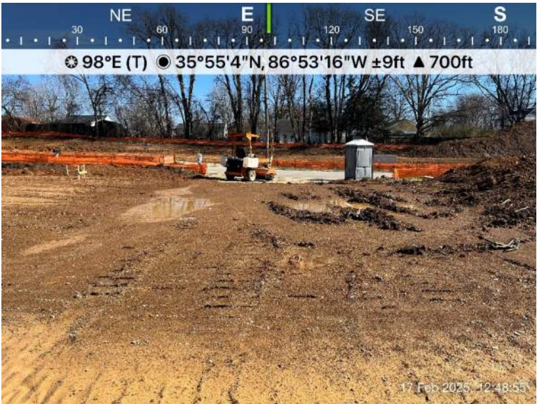
East side of Cherokee site cut to subgrade, street sweeper on site
