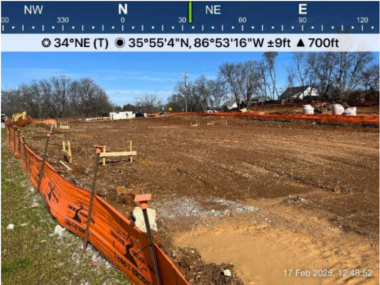
Building pad cut to subgrade
