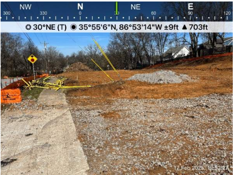
View of driveway at second construction entrance on Shawnee site
