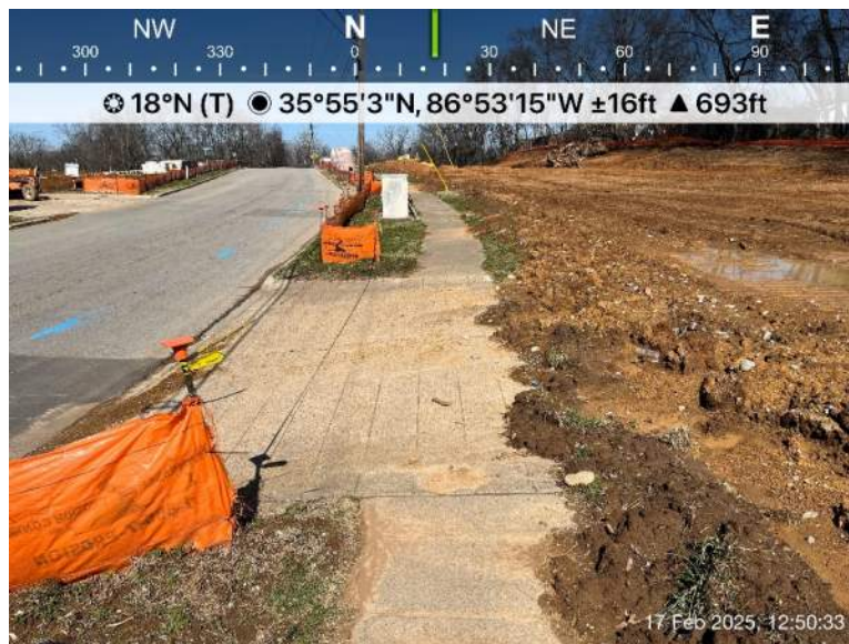
View of Shawnee site and need for silt fence at back of sidewalk at existing driveway entrance
