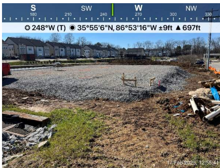
View of building pad T1 at Chickasaw Street on Cherokee site
