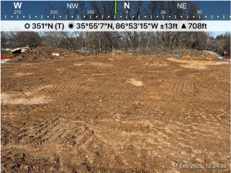
View of Cherokee Building L pad cut to subgrade
