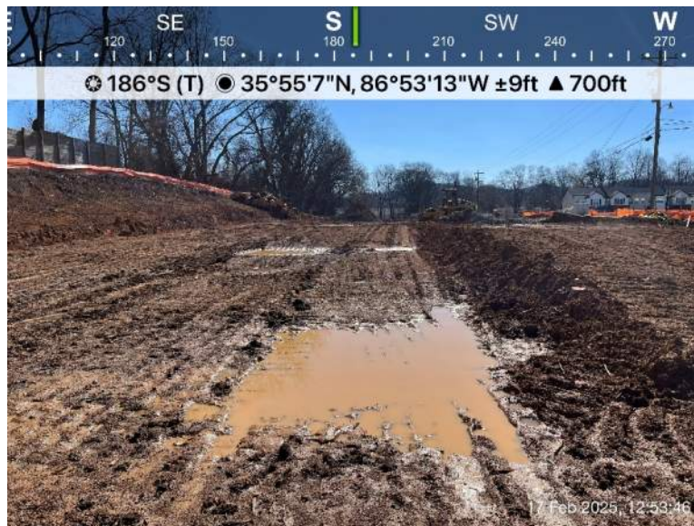
View of Shawnee site cut to subgrade with standing water
