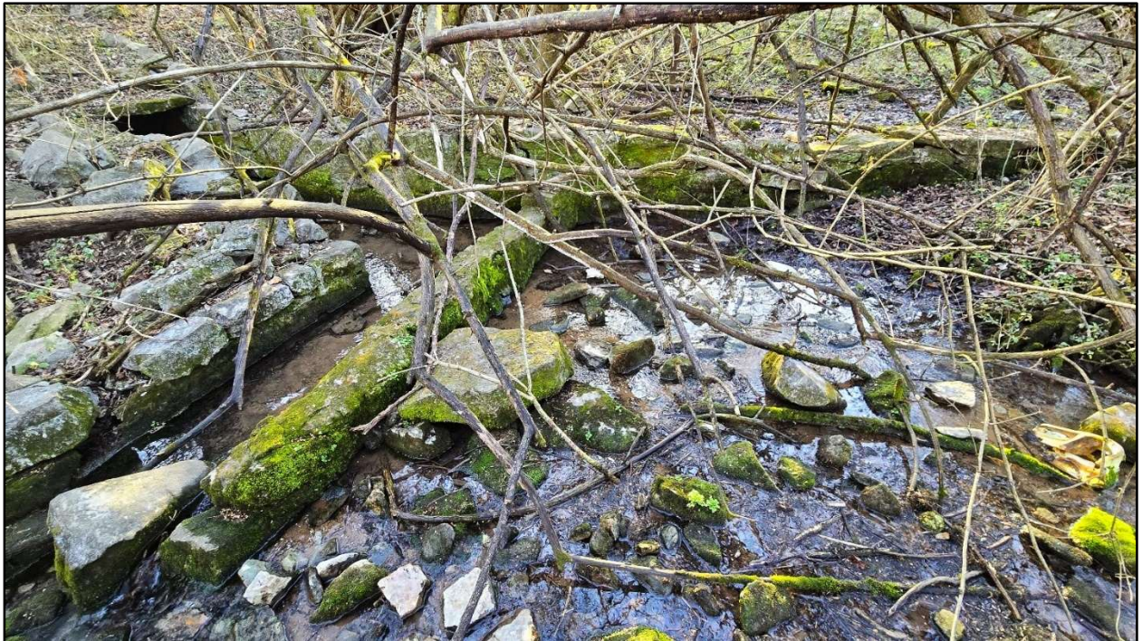
Figure 27. Photograph of the stone cistern discharge looking northwest, February 2025.
