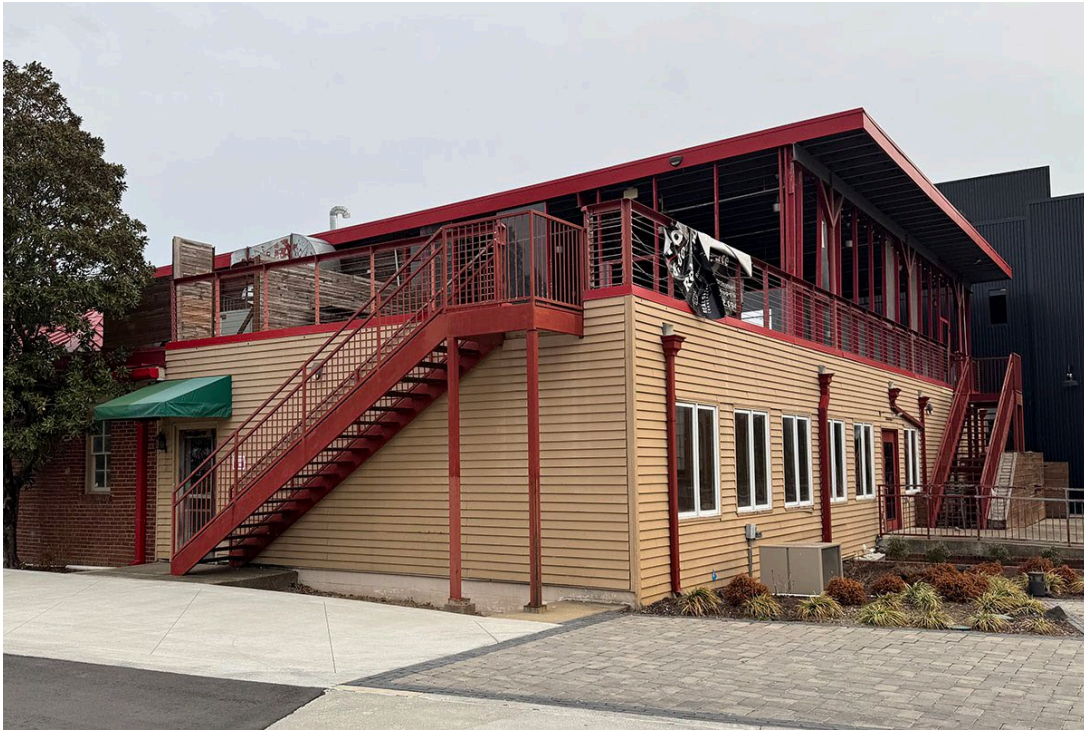
View of Second Floor Patios
