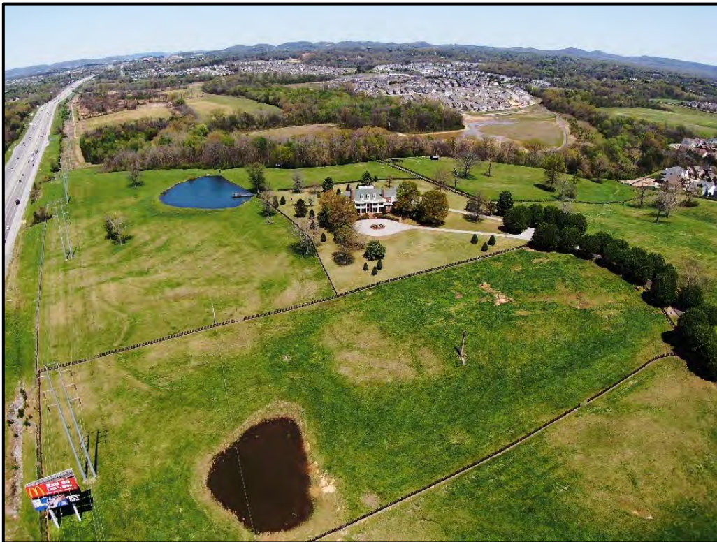
VIEW ALONGSIDE I-65 AND LOCATION OF PROPOSED UTILITY EASEMENT
