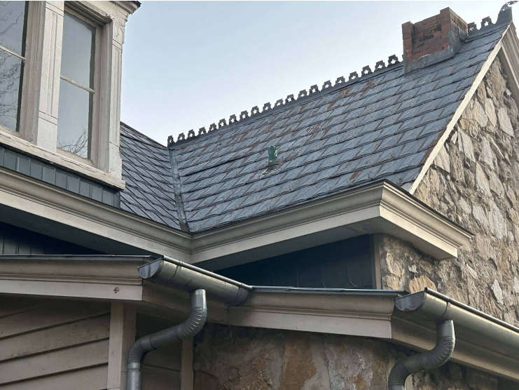
PREVIOUSLY REPLACED REAR TRIM
