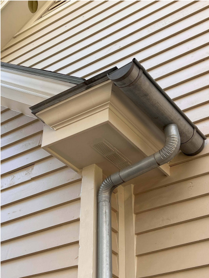
PREVIOUSLY REPLACED TRIM
