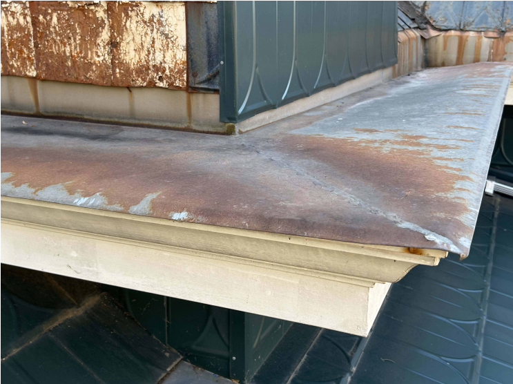
MIX OF METAL SHINGLES AT REAR DORMER
