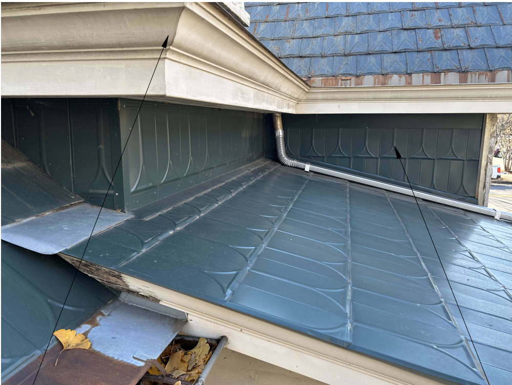
PREVIOUSLY APPROVED REPLACEMENT METAL ROOF
