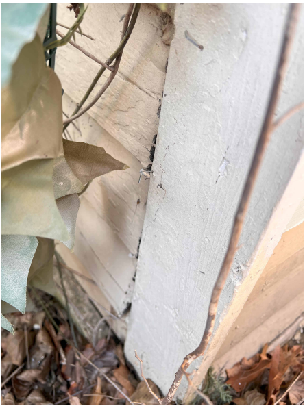
DETERIORATED SIDING
