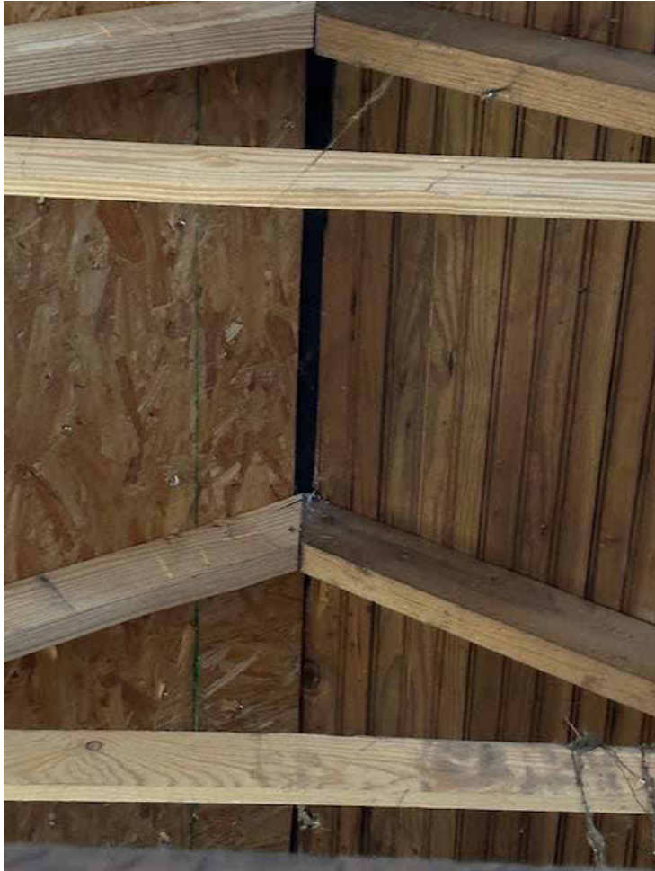
GARAGE CEILING CONSTRUCTION
