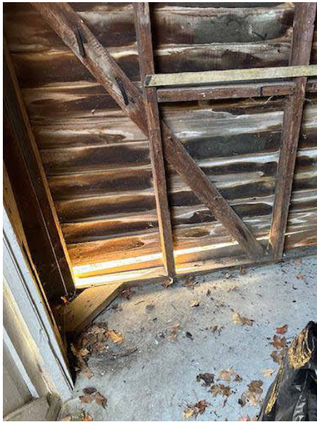
DETERIORATED SIDING
