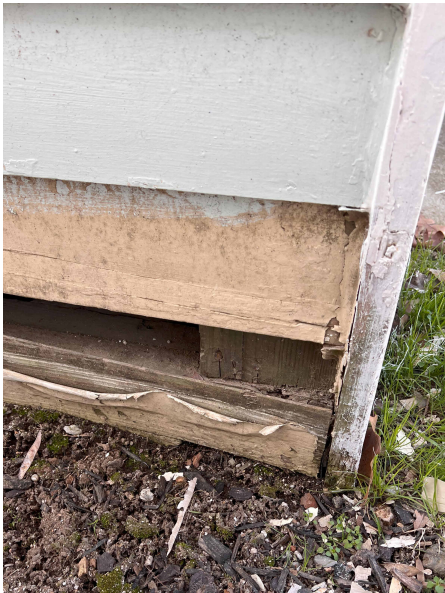
DETERIORATED SIDING
