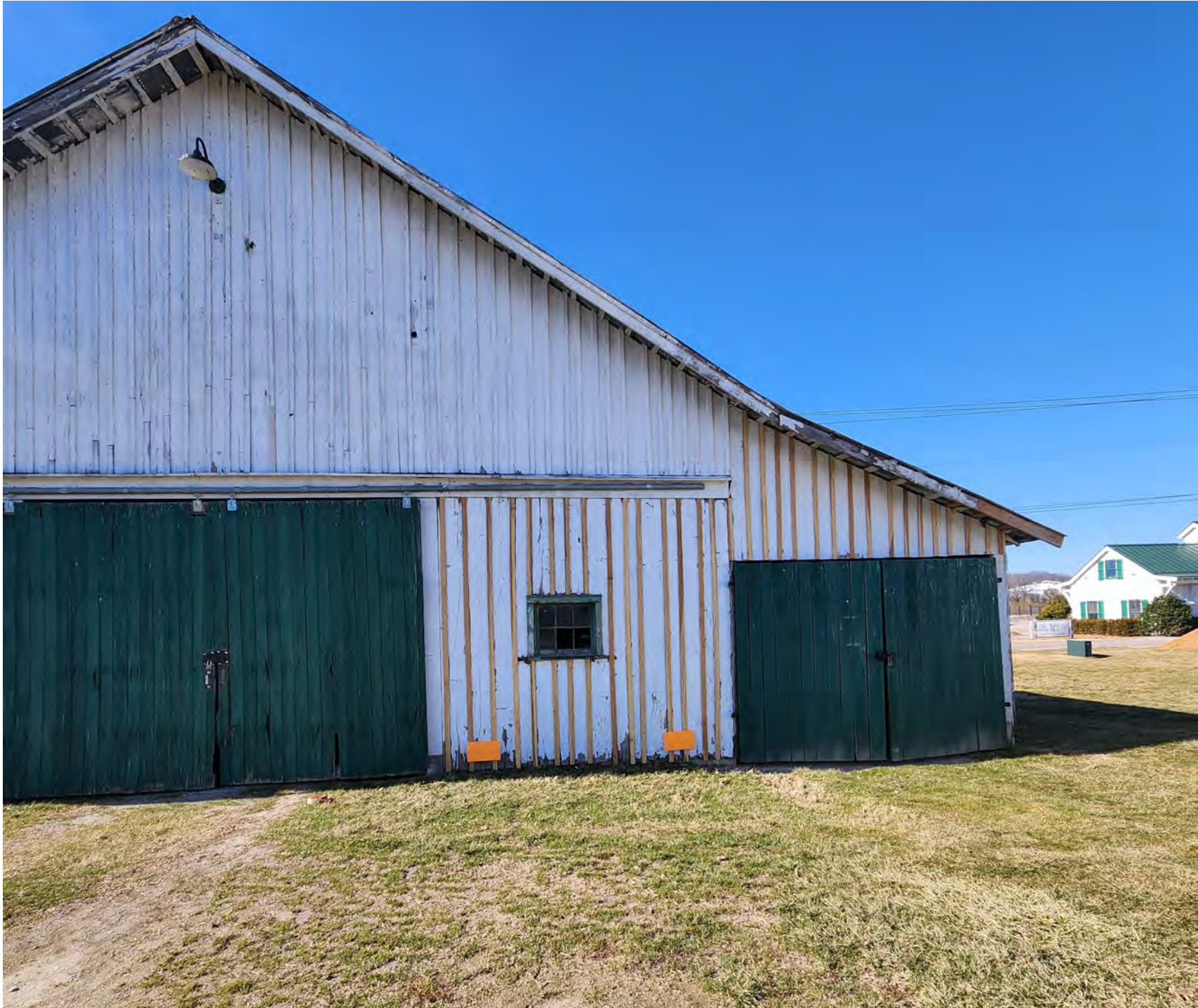
Photo 6: Eastern side of Building A.
