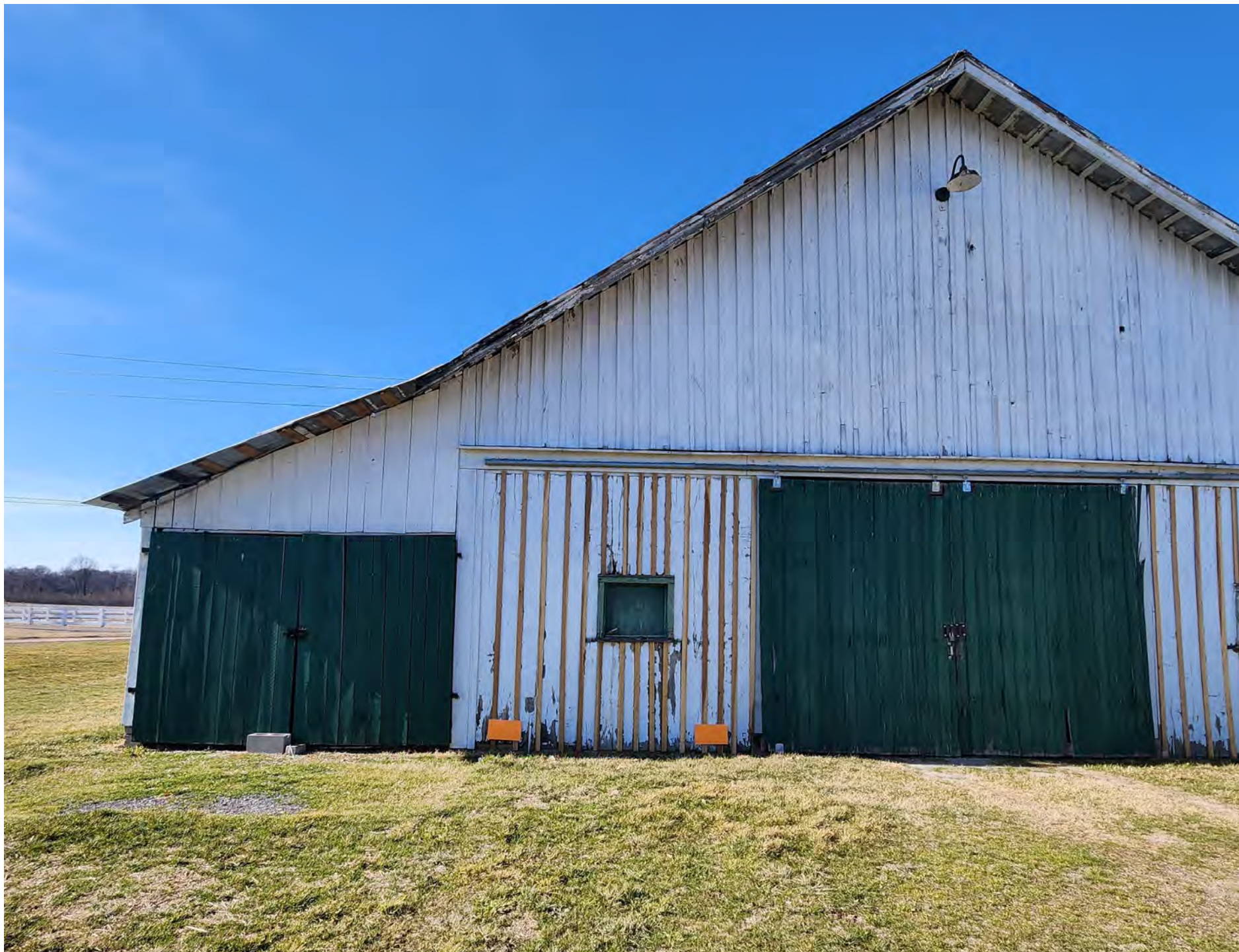
Photo 6: Eastern side of Building A.
