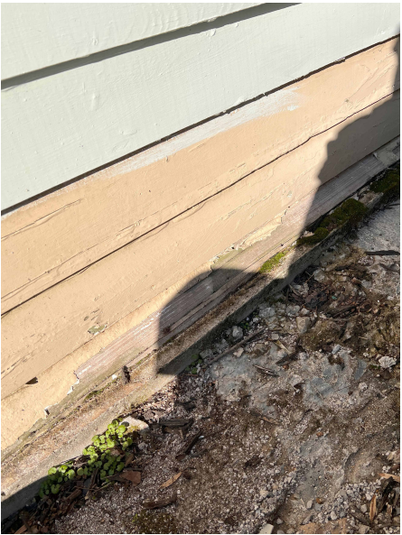
DETERIORATED SIDING
