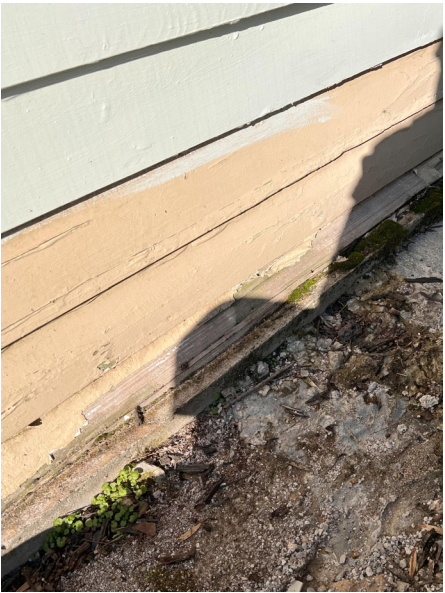
DETERIORATED SIDING
