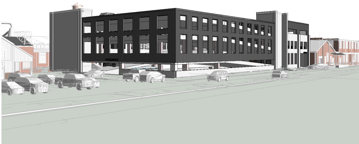
CONCRETE + METAL PANEL 'WINDOW' OPENINGS
