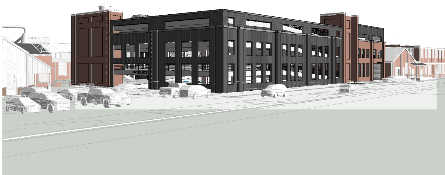
BRICK + METAL PANEL 'WINDOW' OPENINGS
