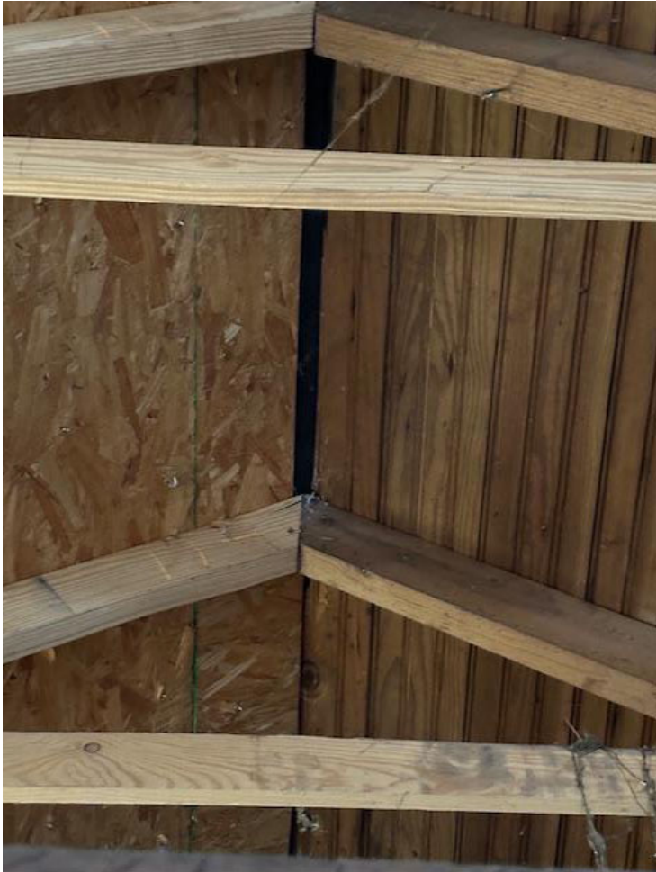
GARAGE CEILING CONSTRUCTION
