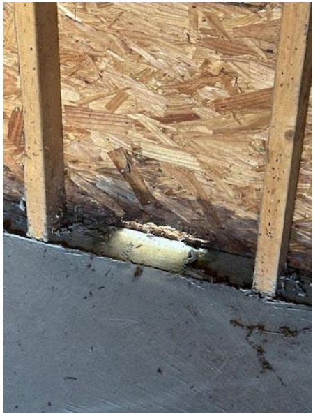
DETERIORATED SIDING
