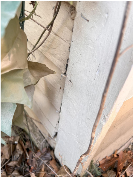
DETERIORATED SIDING
