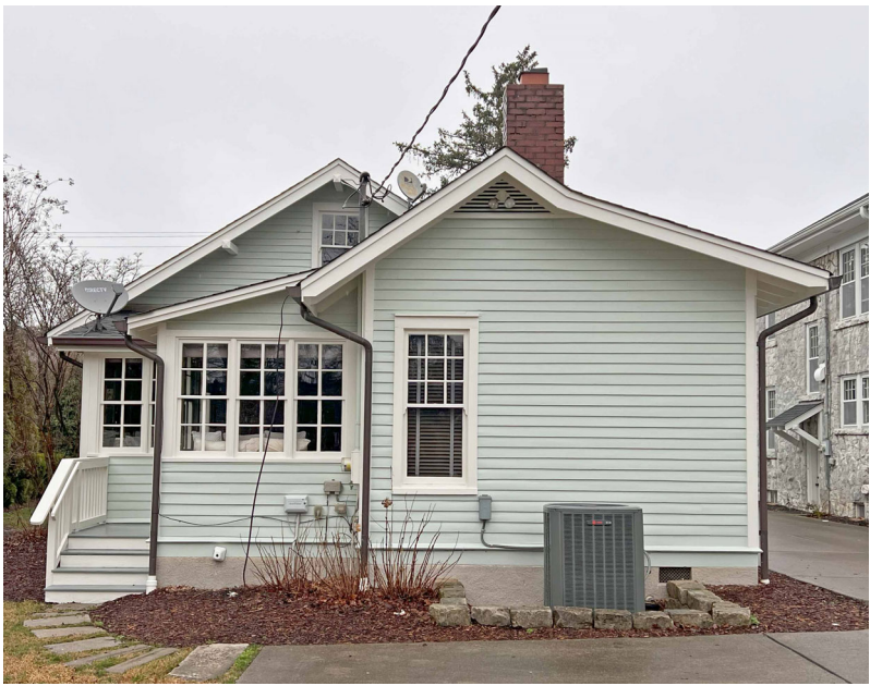
REAR OF EXISTING HOUSE
