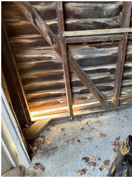
DETERIORATED SIDING
