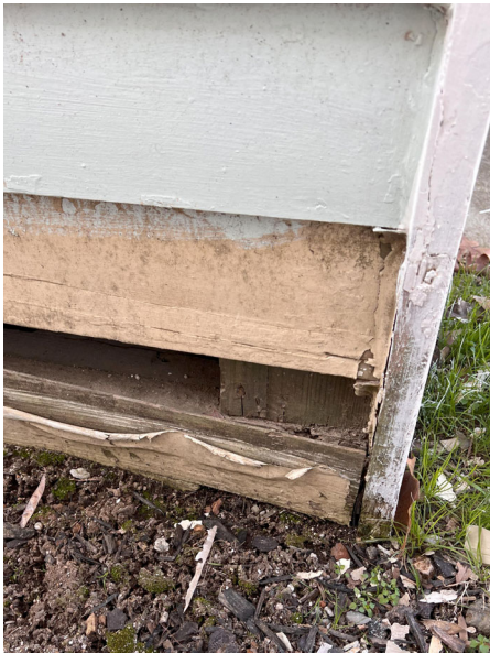
DETERIORATED SIDING
