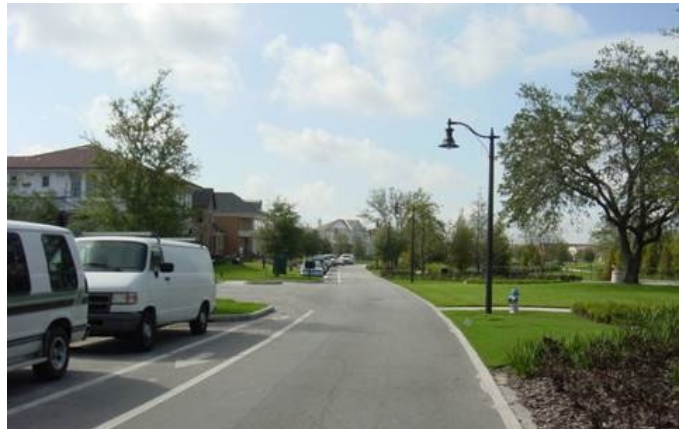
The addition of a bike lane and a parking lane on this street helps to create a narrow travel lane for motorists. (Source: Google)
