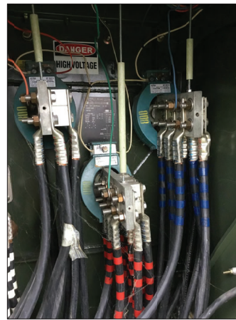
TYPICAL STACKED LUG INSTALLATION
