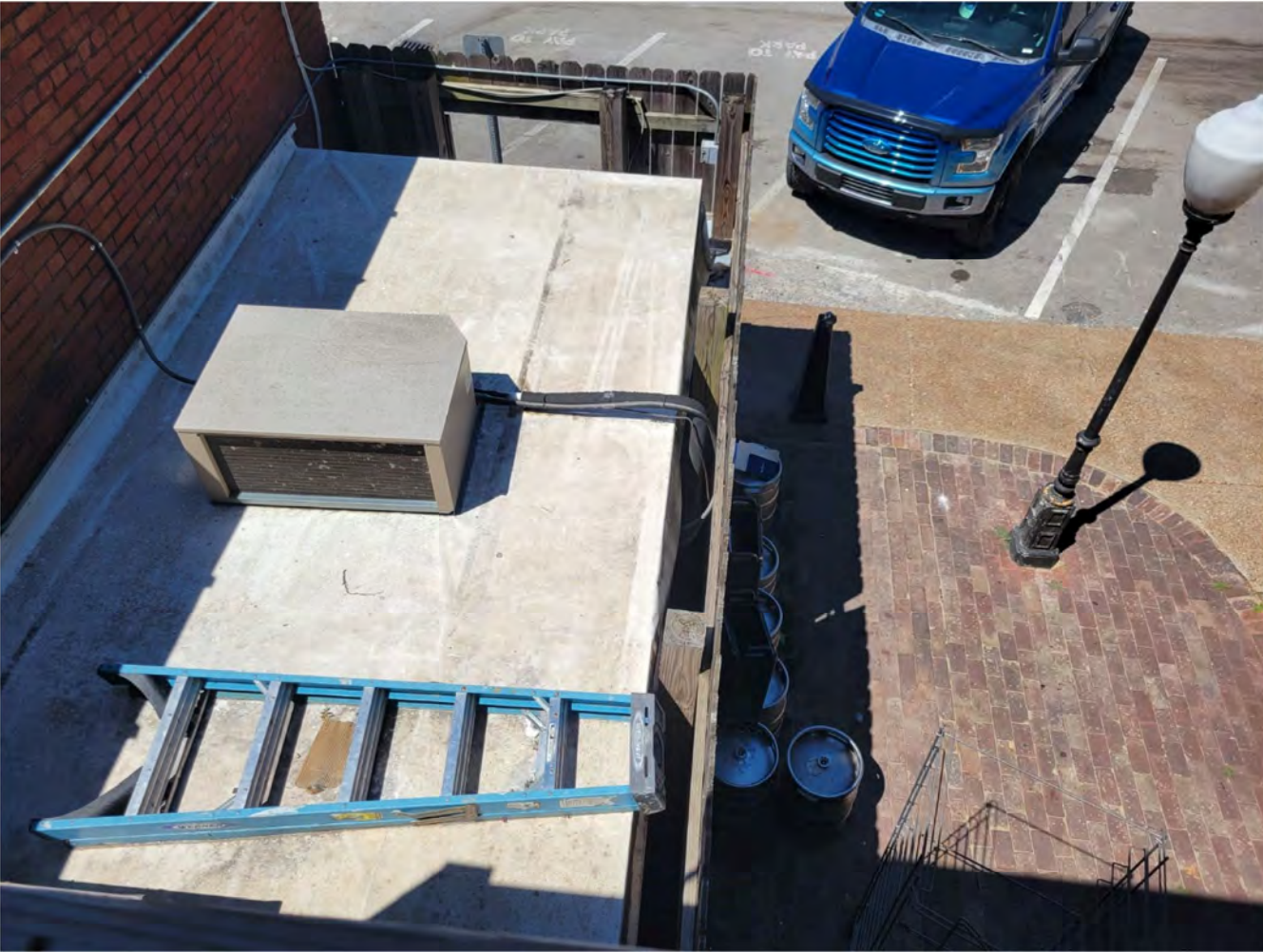
EXISTING CONDITIONS - PHOTO 2
