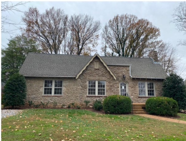
109 Winslow Road/ 2 houses to the left of 115
