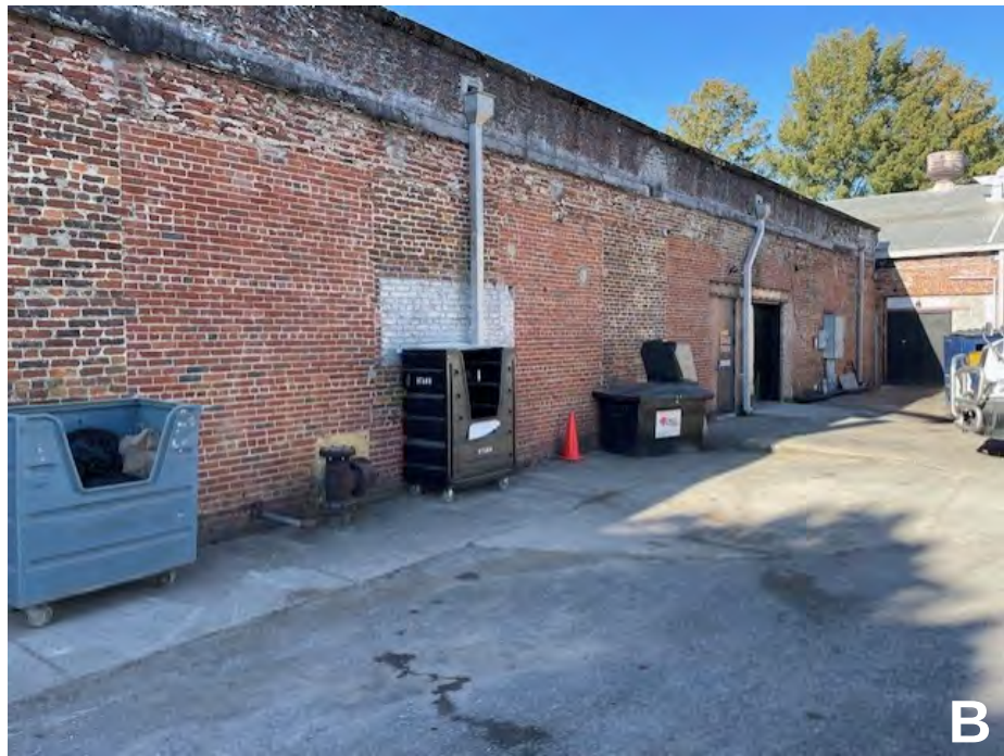
EXISTING BRICK WALLS AT BUILDINGS 3 & 5 HAVE A 2-HR RATING ALL EXISTING DOORS AT THE BACKS OF BUILDINGS 3 & 5 (ADJACENT TO NEW PARKING GARAGE) TO BE UPDATED TO COMPLY WITH A 2-HR WALL RATING. REPLACED DOORS WILL BE SIMILAR IN APPEARANCE TO EXISTING.
