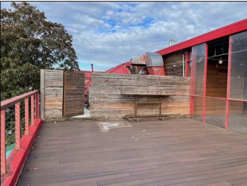
EXISTING - WOODEN MECHANICAL SCREEN
