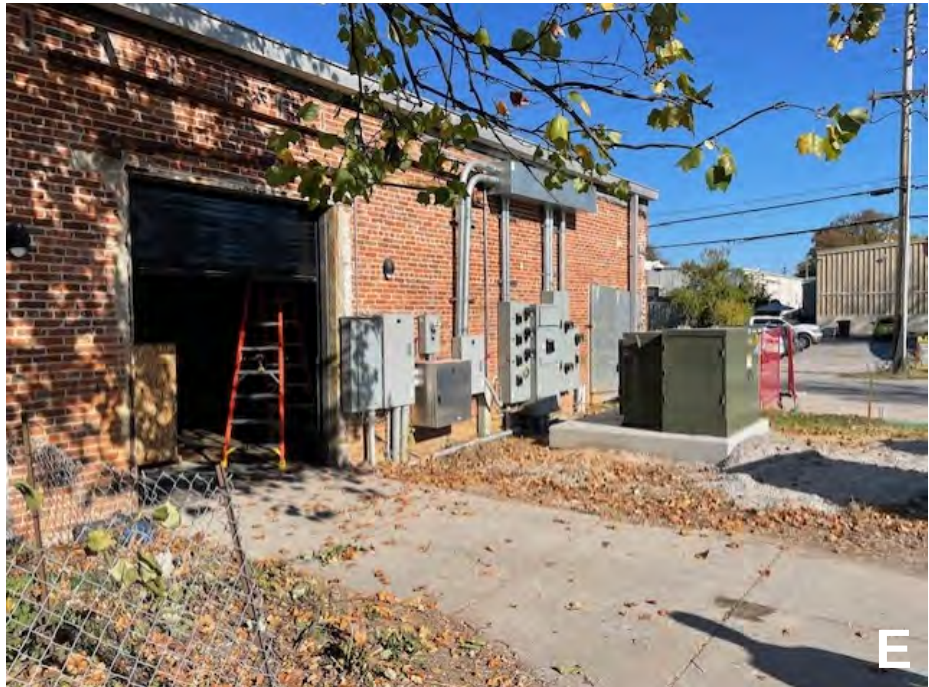
EXISTING BRICK WALLS AT BUILDINGS 3 & 5 HAVE A 2-HR RATING ALL EXISTING DOORS AT THE BACKS OF BUILDINGS 3 & 5 (ADJACENT TO NEW PARKING GARAGE) TO BE UPDATED TO COMPLY WITH A 2-HR WALL RATING. REPLACED DOORS WILL BE SIMILAR IN APPEARANCE TO EXISTING.
