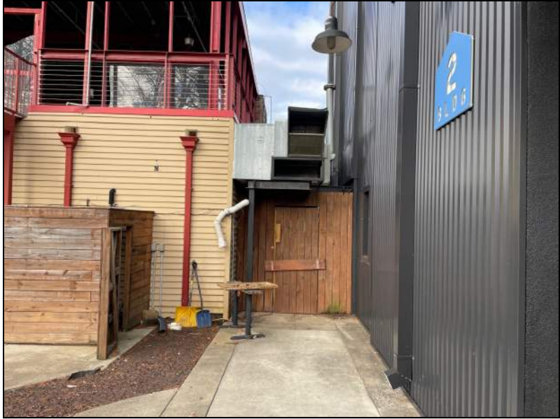
EXISTING HVAC EQUIPMENT TO BE REMOVED
