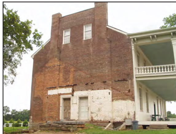
Archeological work has been conducted recently at Carnton Plantation in the vicinity of the former kitchen wing. Serving as the original section of the house, it was destroyed years ago by a tornado, but the "ghost" of its end wall is visible on the facade shown above.
