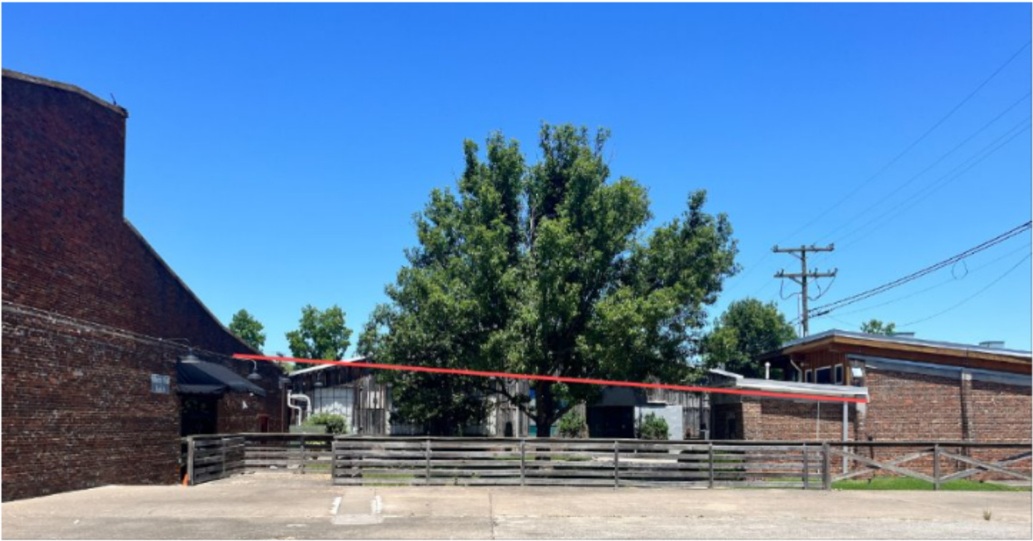
Estimated roofline lines up with color and brick change on Building 12. It's believed that the change is the difference between exterior and interior brick. The darker bricks on Building 12 are more uniform and smooth, while the bricks on the lower portion of Building 12 and on Building 10 are rougher, lighter, and less uniform, indicating an interior origin.
