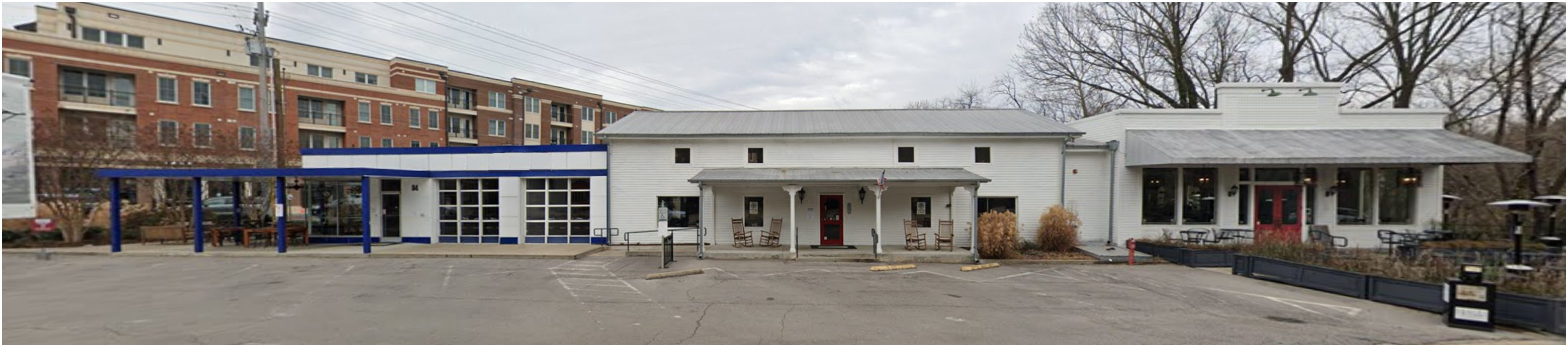
EXISTING FRONT FACADE
