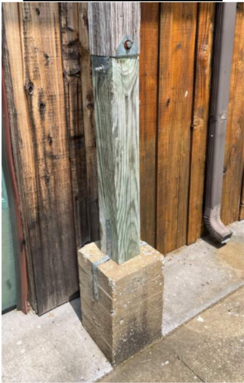
Photo 4 (typical exterior column repair)
