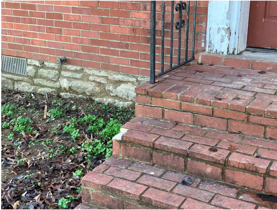
VIEW OF EXISTING LIMESTONE FOUNDATION
