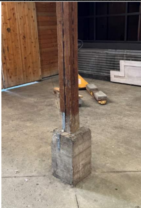
Photo 1 (typical interior column base condition)
