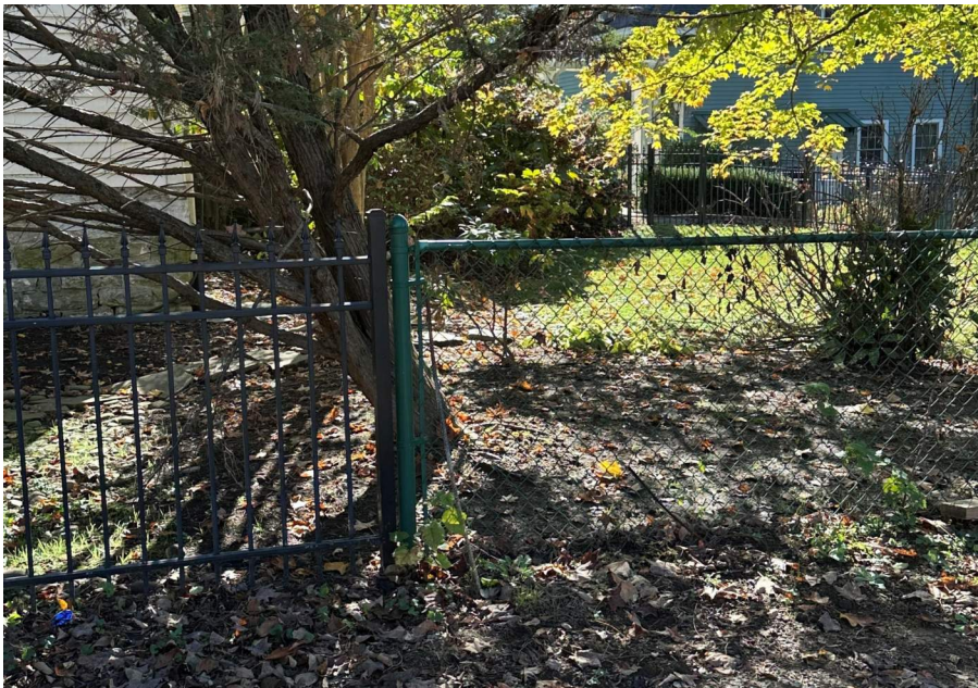
EXISTING IRON FENCE AND CHAIN LINK CONNECTION AT ADJACENT PROPERTY TO THE LEFT
