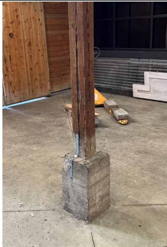
Photo 1 (typical interior column base condition)
