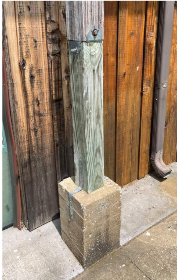
Photo 4 (typical exterior column repair)
