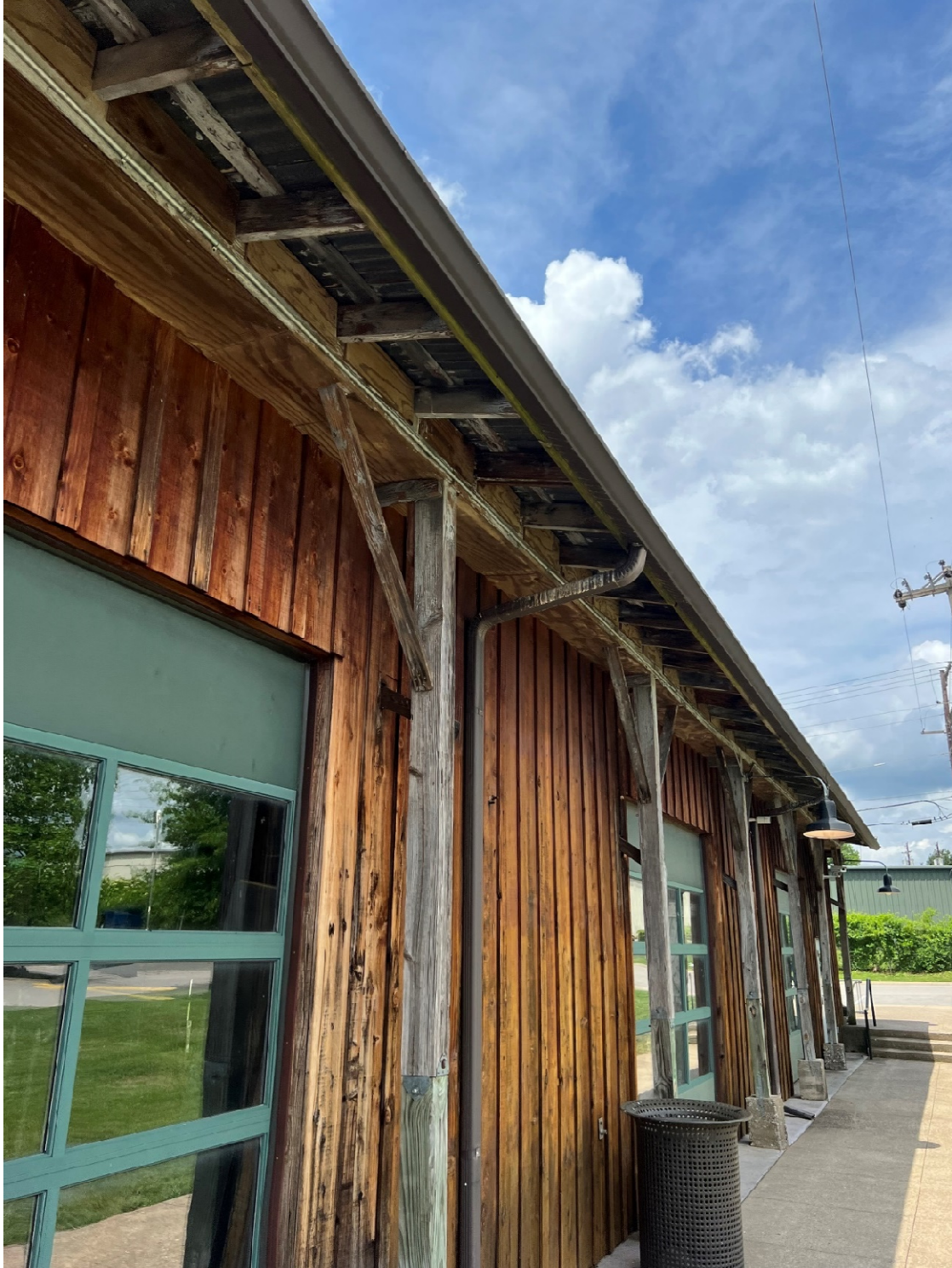
View at southeast eaves and column line
