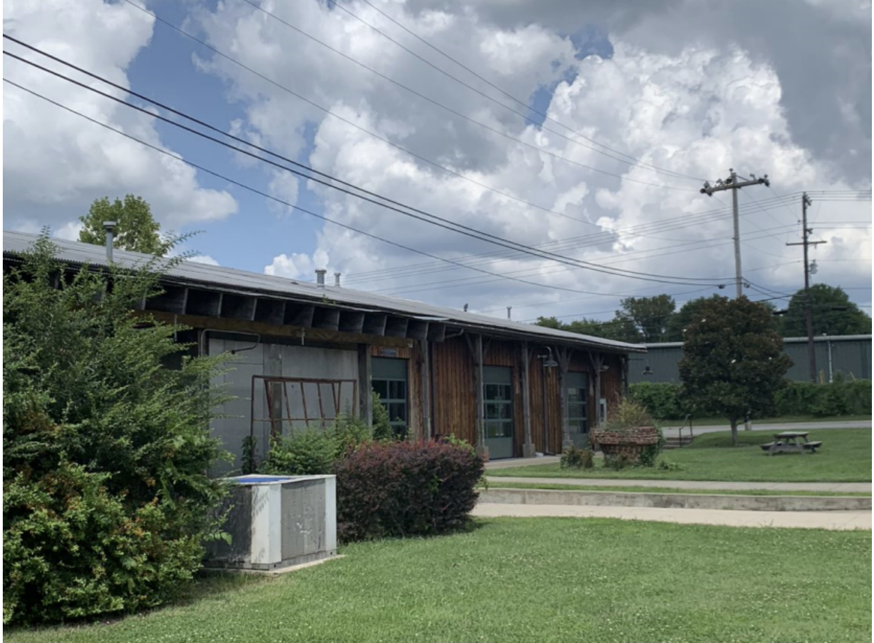
View from southeast side of site
