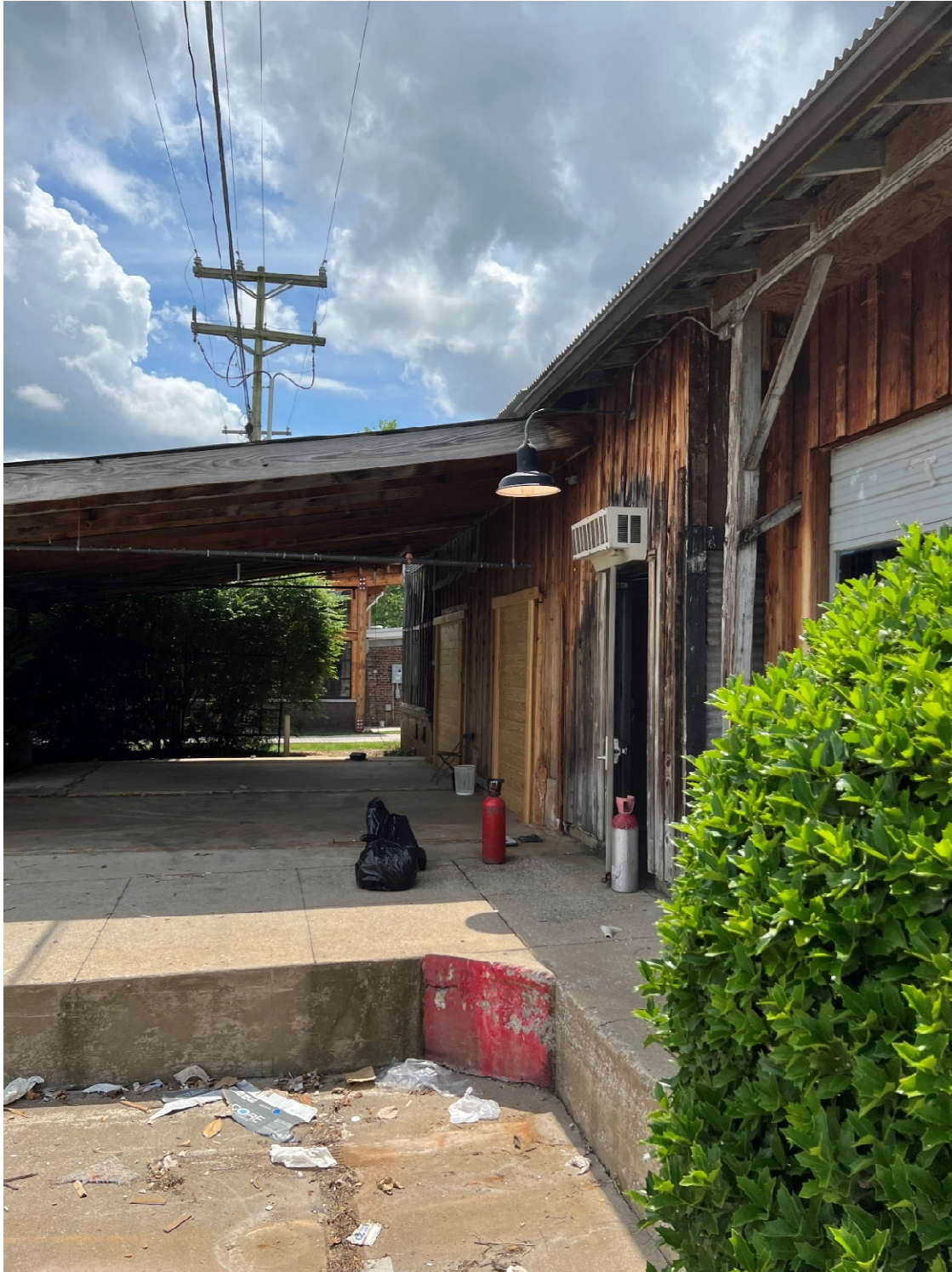
East elevation looking south
