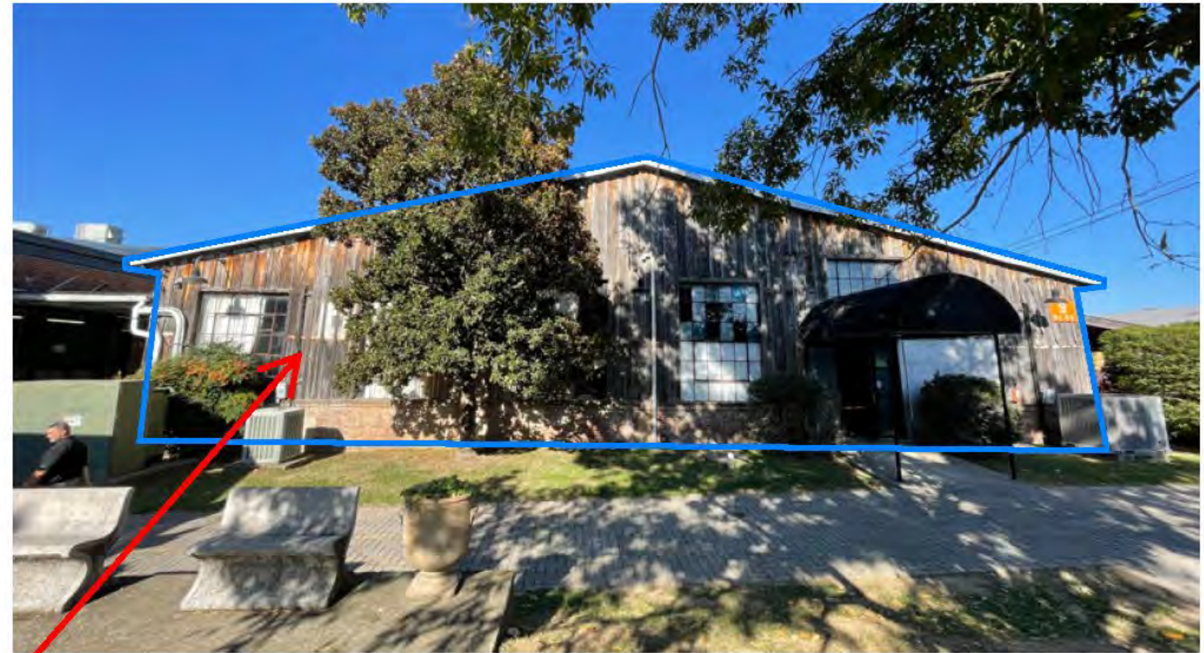
Inferior views from eastern parking lot. Front bay & ~50% of the footprint to remain. Courtyard design will utilize the existing column grid, and any historic heavy timber will be incorporated into the new courtyard (non-structurally) as allowed by code.
