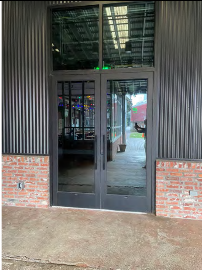
EXISTING STOREFRONT AT B5
