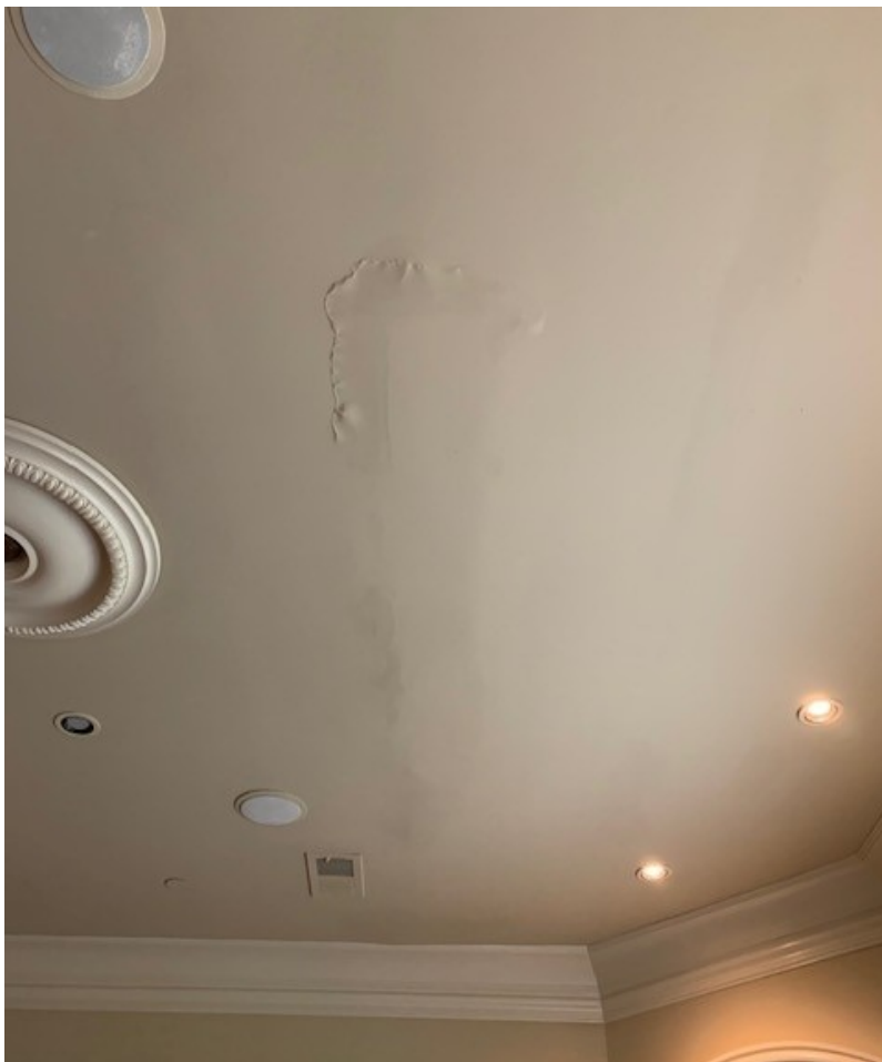
DAMAGE CAUSED BY LEAK FROM PATIO DOORS & THRESHOLD ABOVE
