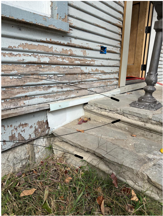
FRONT ENTRY STEPS
