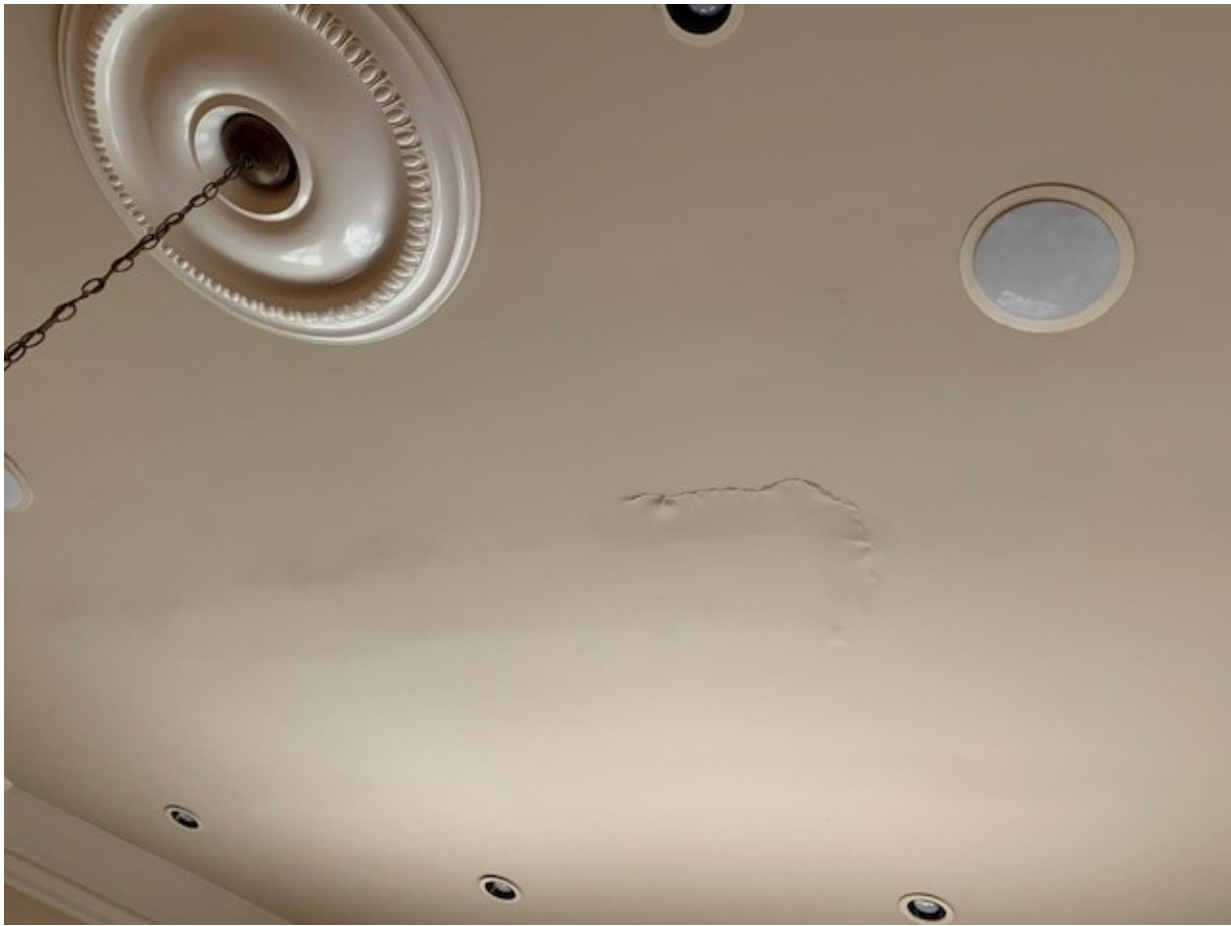
DAMAGE CAUSED BY LEAK FROM PATIO DOORS & THRESHOLD ABOVE
