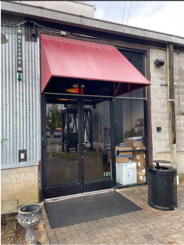
EXISTING STOREFRONT AT B12
