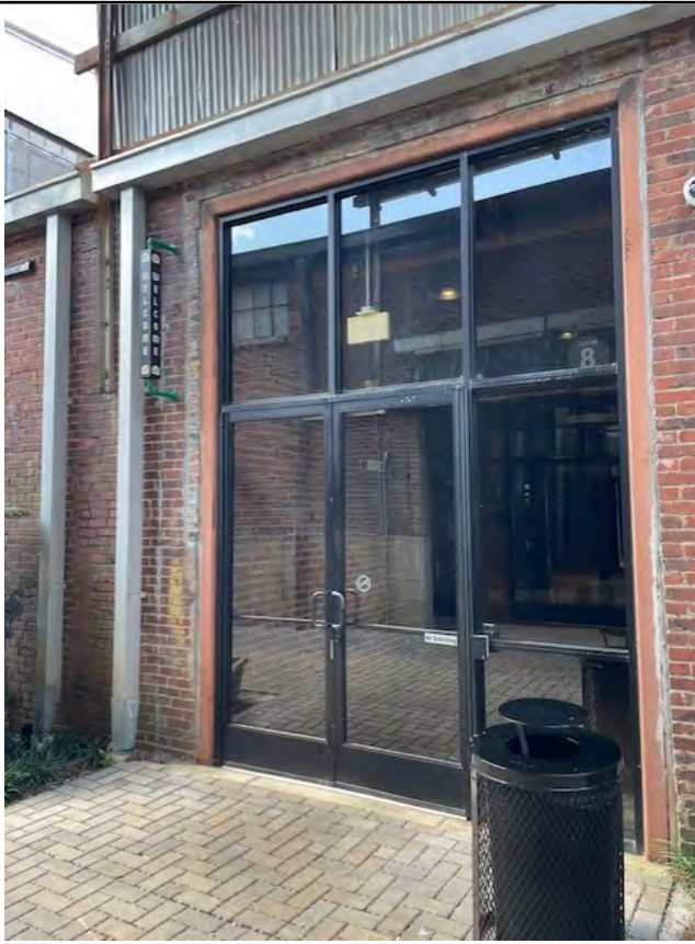
EXISTING STOREFRONT AT B11
