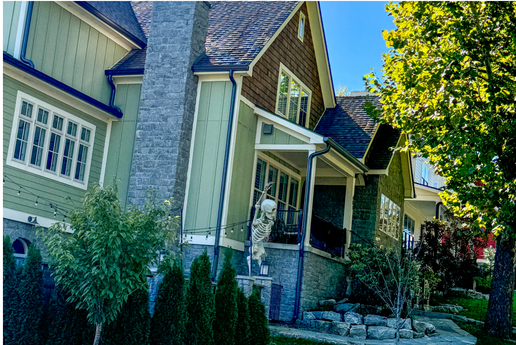
Side of home showing fence covered by trees.
