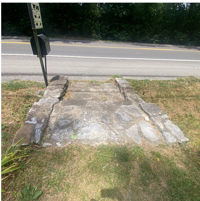
Existing stone stairs and mailbox on site
