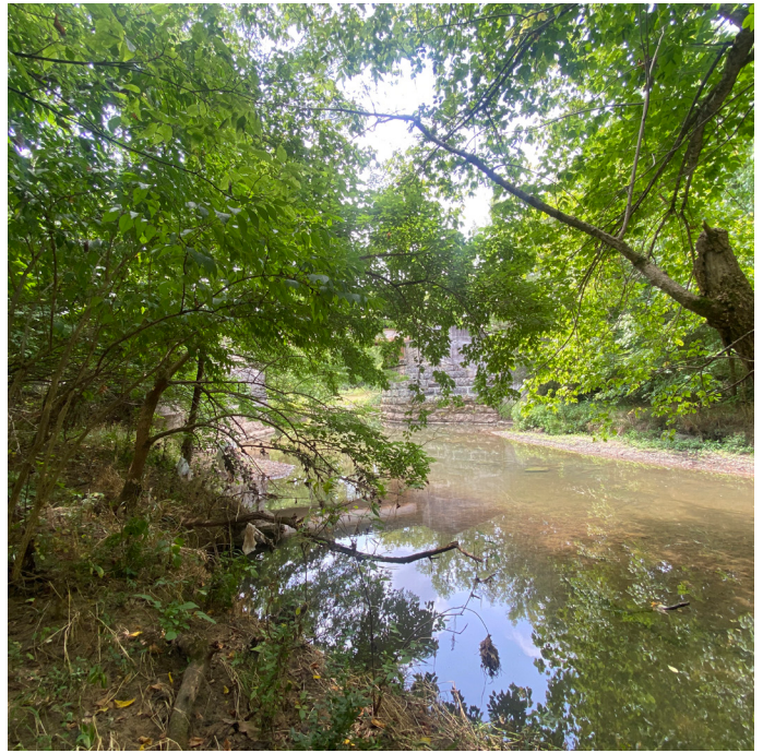
Spencer Creek and existing railroad bridge crossing
