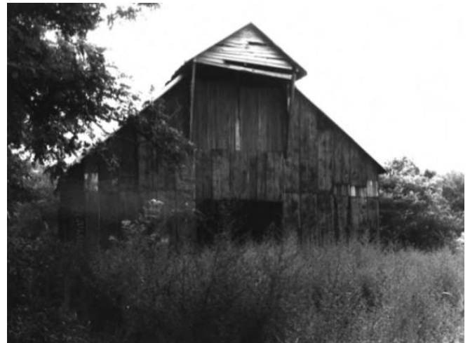
Barn on site, 1987
