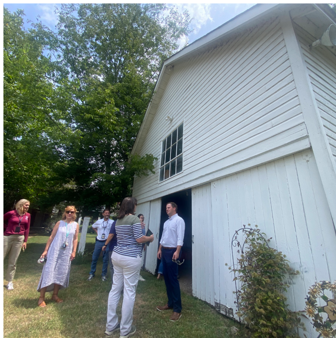
Existing structure on site
