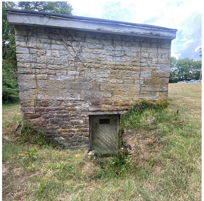
Existing structure on site
