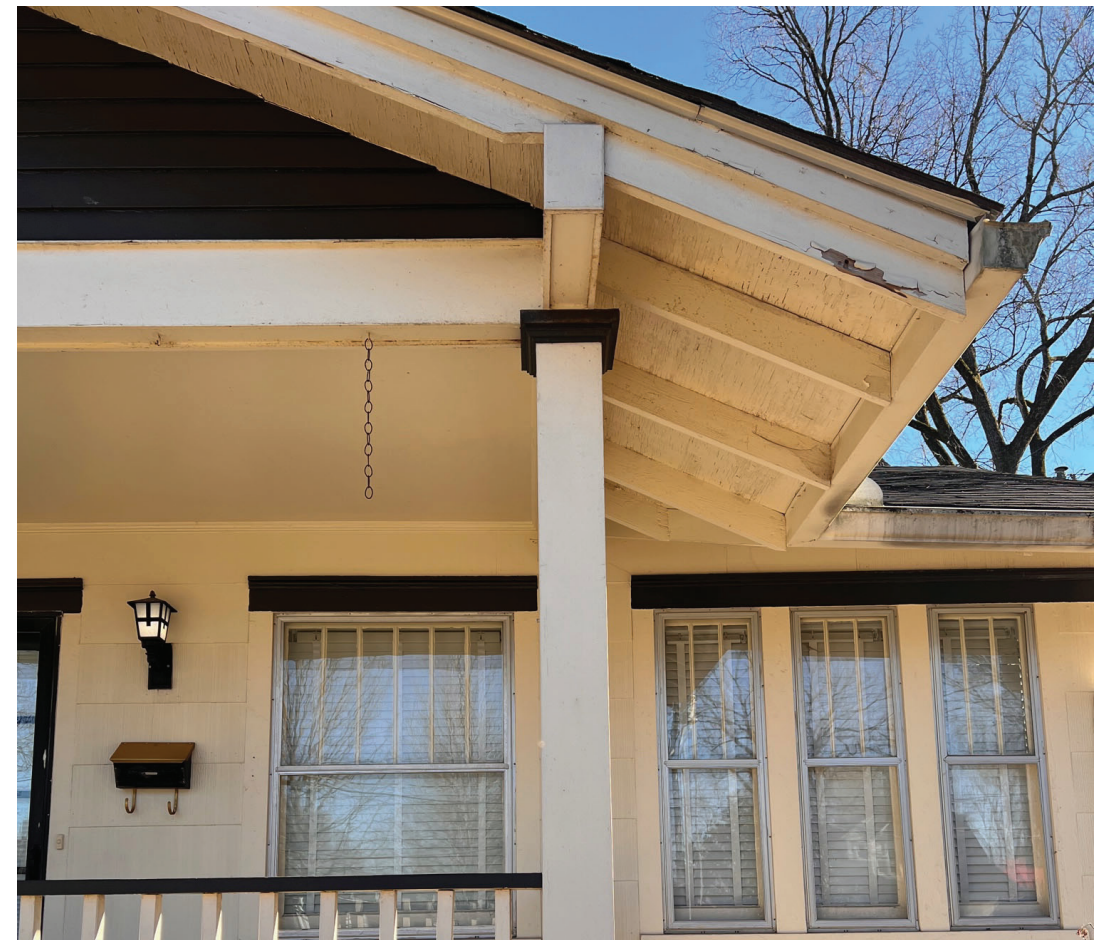
ORIGINAL PORCH ROOF
