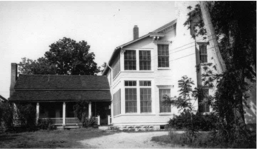
SIDE VIEW - EXISTING ADDITION THAT HAS BEEN DEMOLISHED
