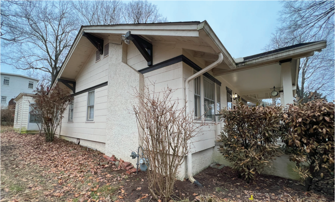
LEFT SIDE GABLE
