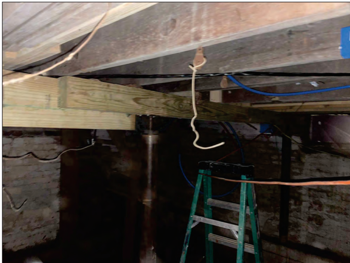
3 Installed supplemental girder is not continuous and is supported on 4x4 post and screw jacks. Replace with a (2) 1 3/4 x 11 7/8 LVL with CMU pier or steel post under the hallway walls as shown on plan.
