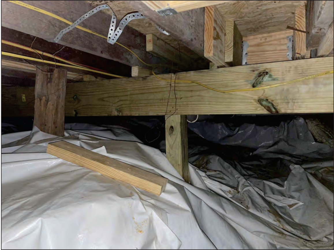
3 Installed supplemental girder is not continuous and is supported on 4x4 post and screw jacks. Replace with a (2) 1 3/4 x 11 7/8 LVL with CMU pier or steel post under the hallway walls as shown on plan.
