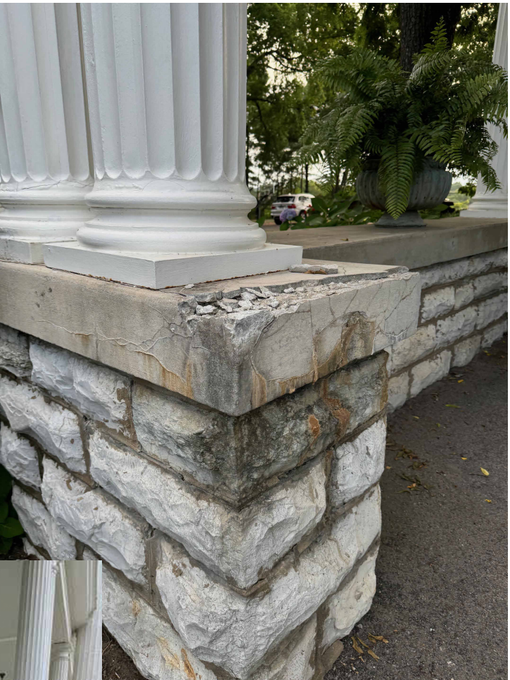
REPAIR DAMAGE TO CONCRETE WALL CAP AT PORTE COCHERE
