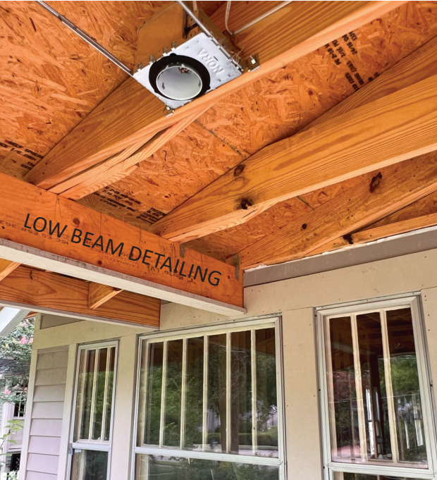
FRONT PORCH DETAIL
