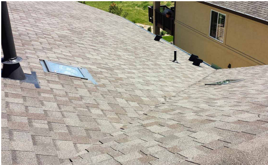
FLAT SUN TUNNEL INSTALLED
