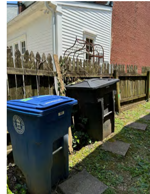
EXISTING FRONT RIGHT • RIGHT PICKET FENCE TO BE REPLACED IN KIND ALONG PROPERTY LINE
