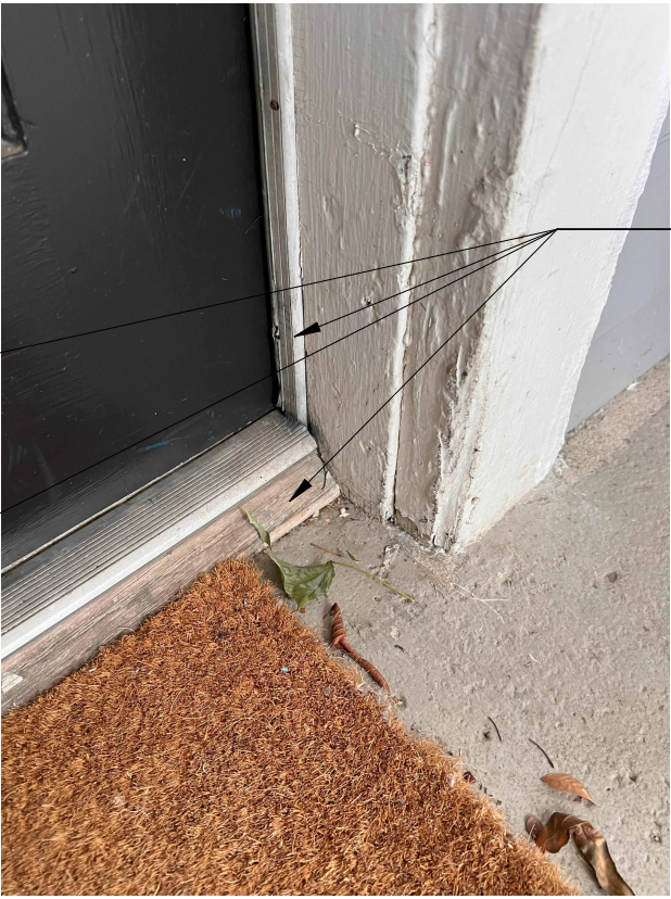
REPLACEMENT SILL AND JAMB TRIM
