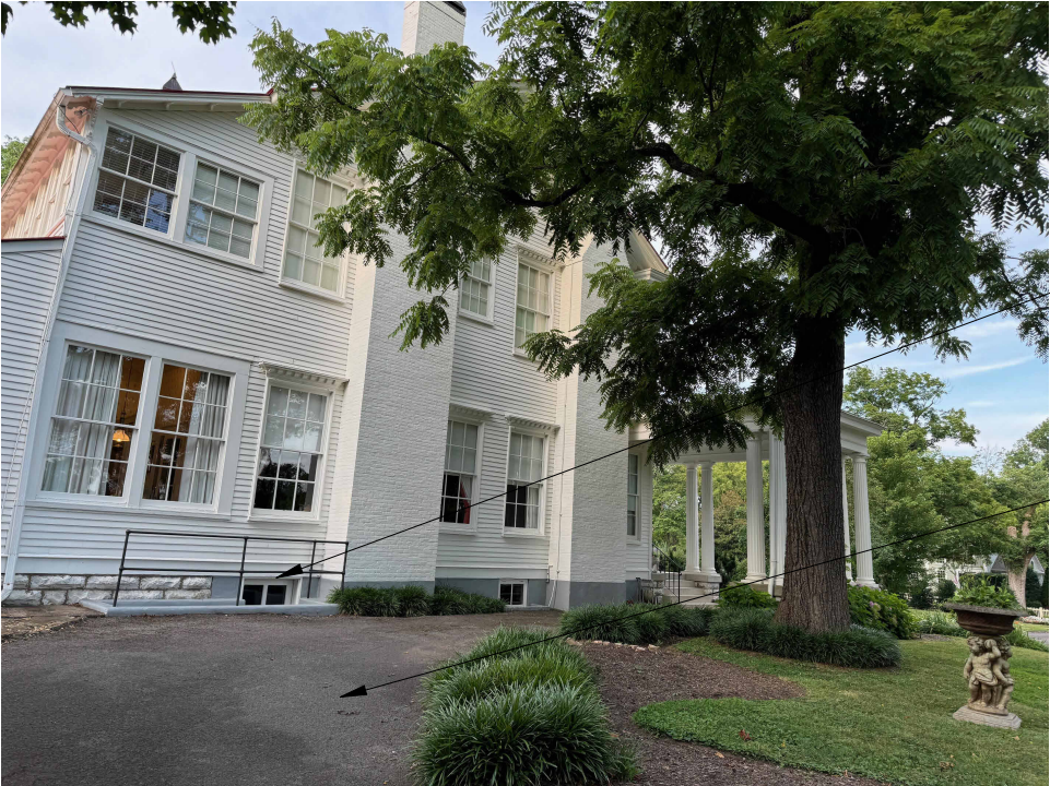
RESIDENCE LEFT SIDE
