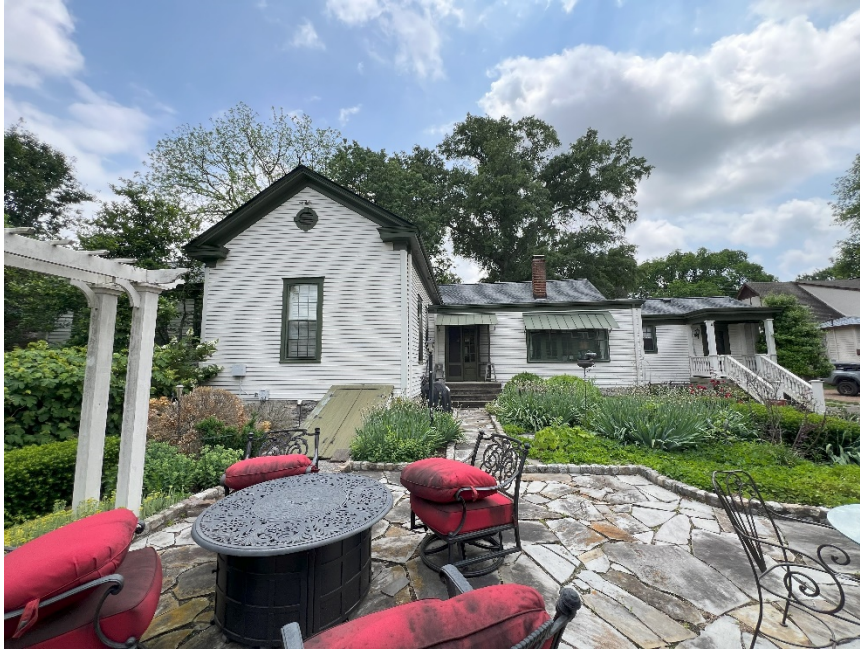
Rear View from Patio
