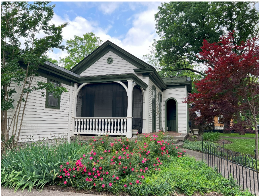
Side View from Driveway
