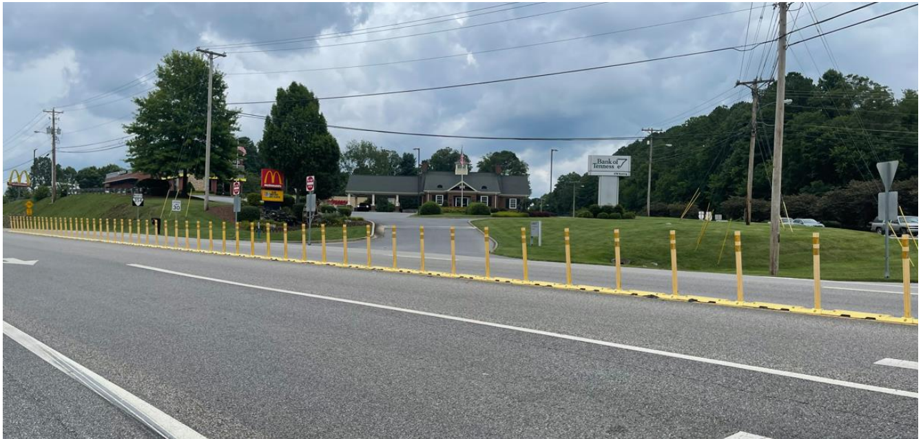
Figure 3 Example of Temporary Curbing with Delineators
