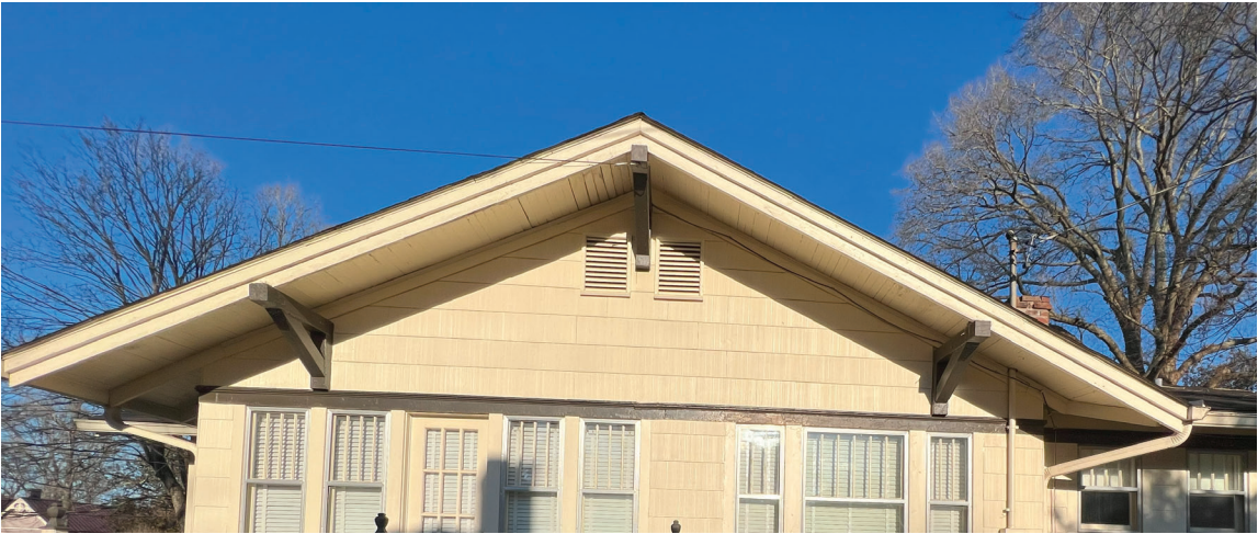
RIGHT SIDE GABLE
