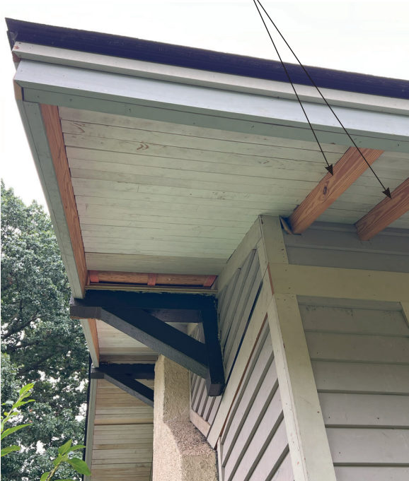
LEFT SIDE GABLE DETAIL
