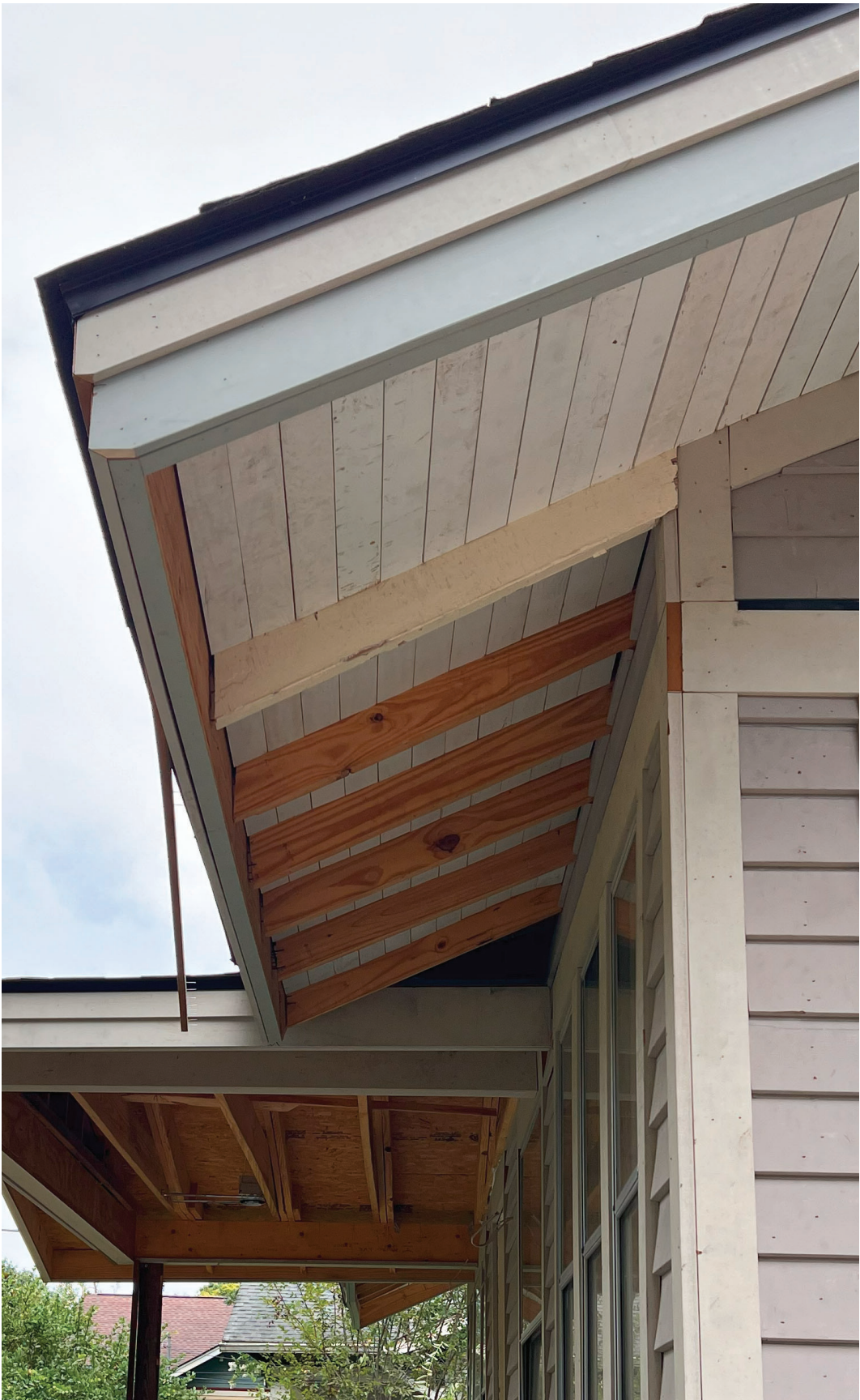
AS-BUILT EAVE & GABLE END CONSTRUCTION
