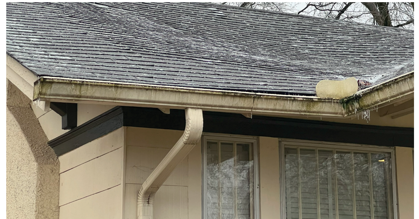
ORIGINAL GUTTER AND RAFTER TAILS
