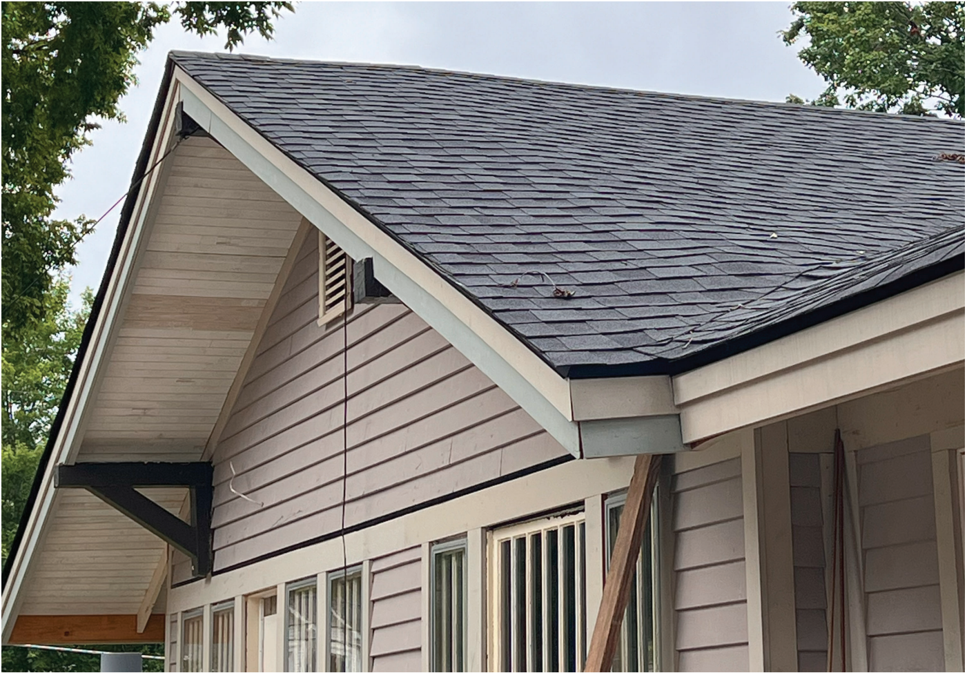
RIGHT SIDE GABLE
