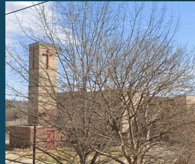
55-foot tower, Lewisburg Pk
