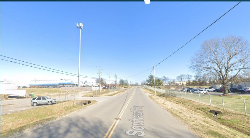
160-foot tower , Southeast Parkway
