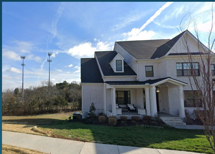
150-foot tower, 3200 Boyd Mill Ave
