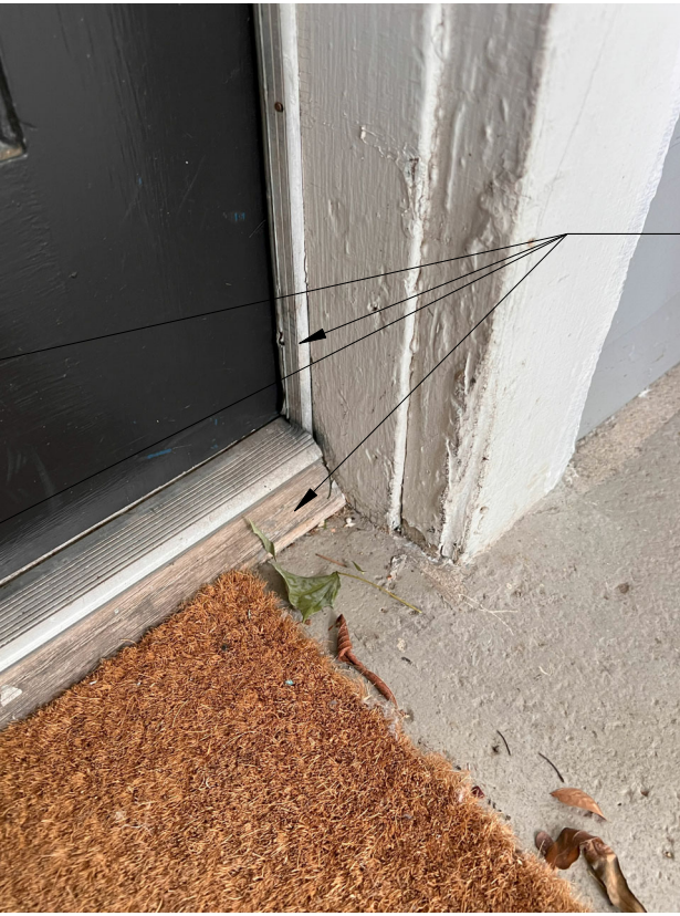
REPLACEMENT SILL AND JAMB TRIM
