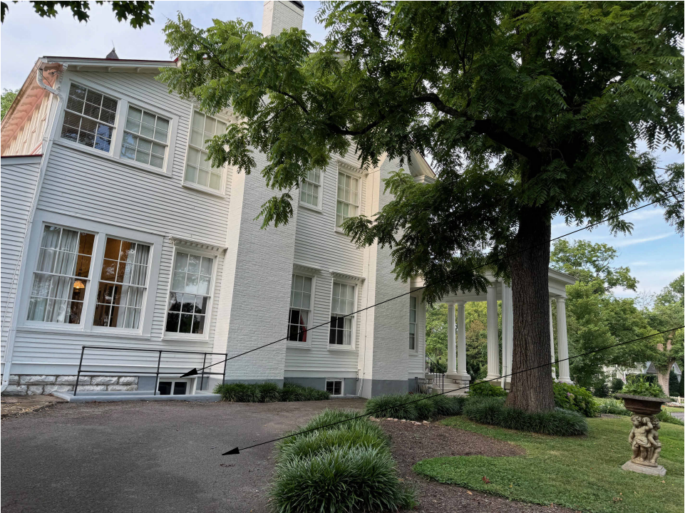
RESIDENCE LEFT SIDE
