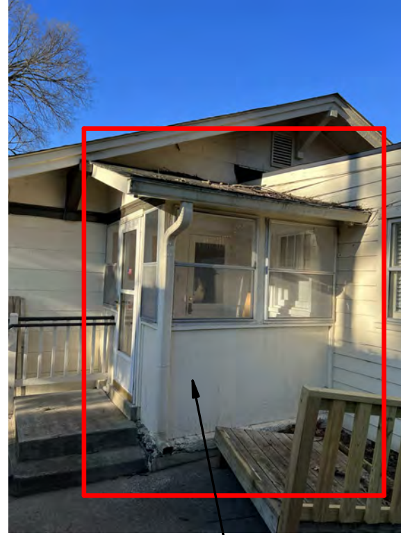
REAR MUDROOM REMOVE REAR MUD ROOM ADDITION AND REAR ENTRY. CONSTRUCT NEW ADDITION. SEE PROPOSED PLANS.
