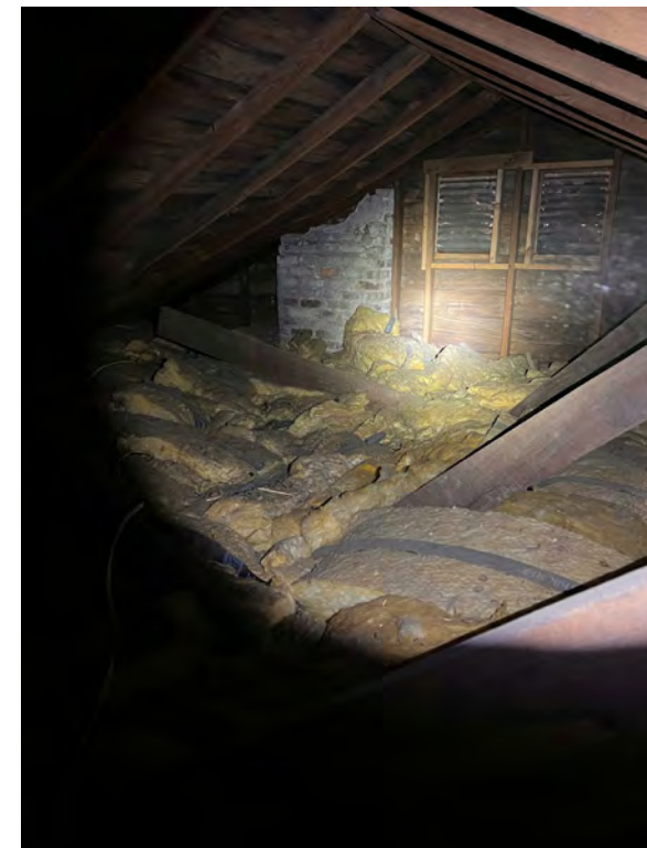
EXISTING CHIMNEY IN ATTIC SHOWING BRICK
