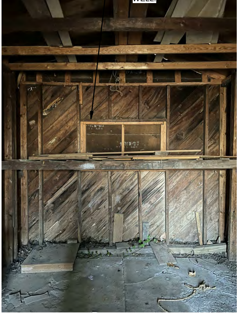
INTERIOR OF RIGHT PORTION OF CARRIAGE HOUSE
