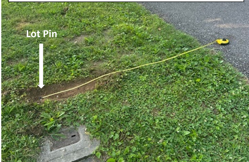
Photo 1: 305 Berry Circle Front Setback pin is approximately 6' from Street Edge
